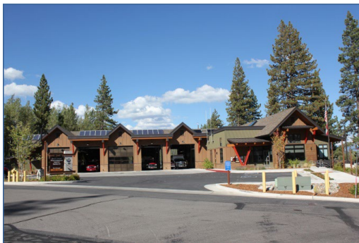
North Tahoe Fire Protection District Headquarters and Station 51 in Tahoe City
