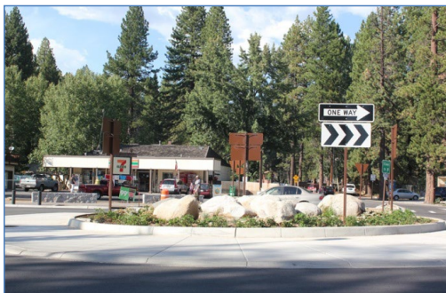
New roundabout in Kings Beach
