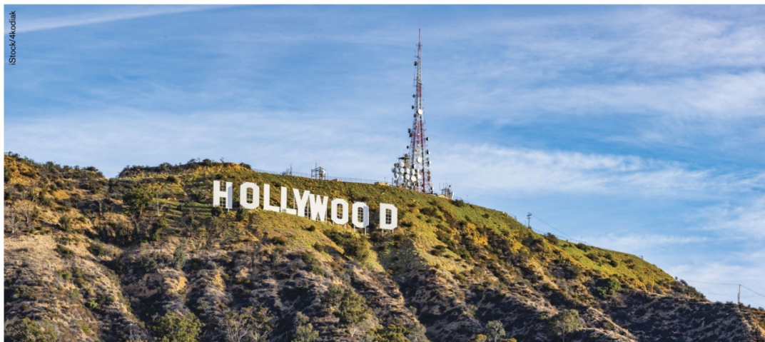
Although towers can alter iconic views, the FCC does not require licensees to consider aesthetic impacts.
