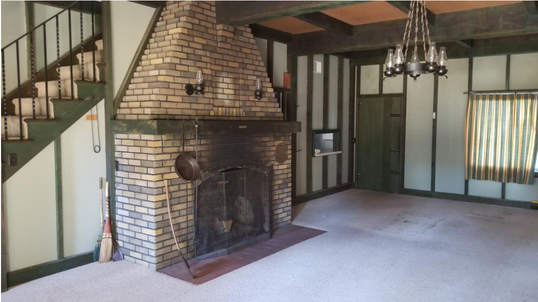
Figure 14. Fireplace in Living/Dining Room (Looking northwest)
