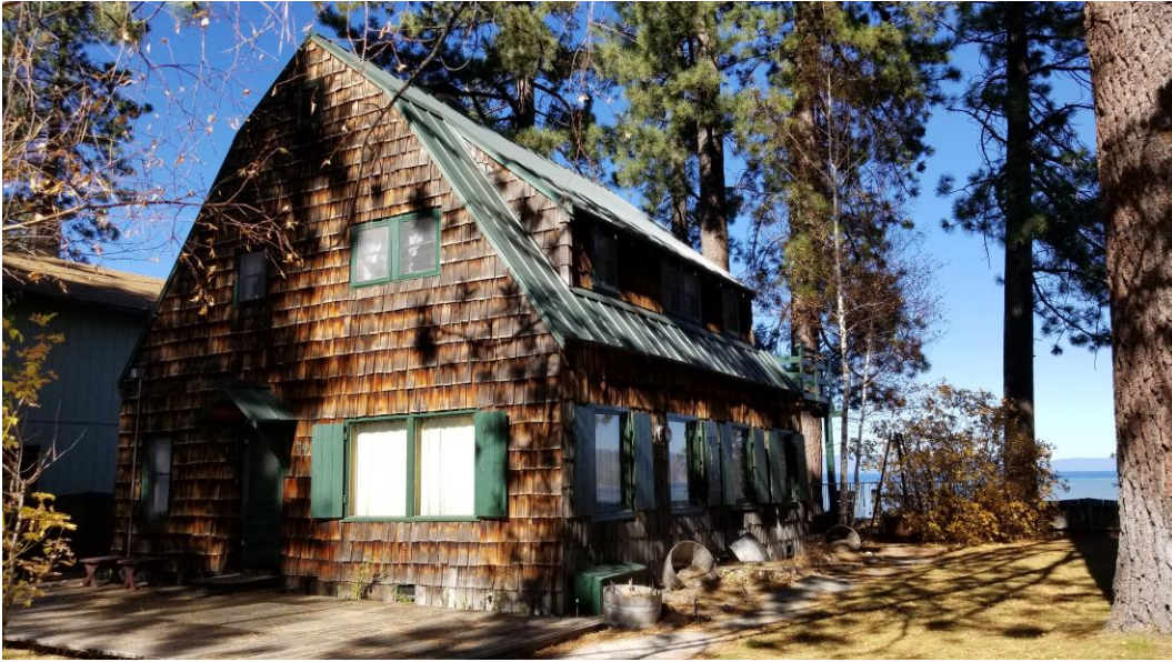
Figure 10. Southeast Corner of Cabin (Looking northwest)
