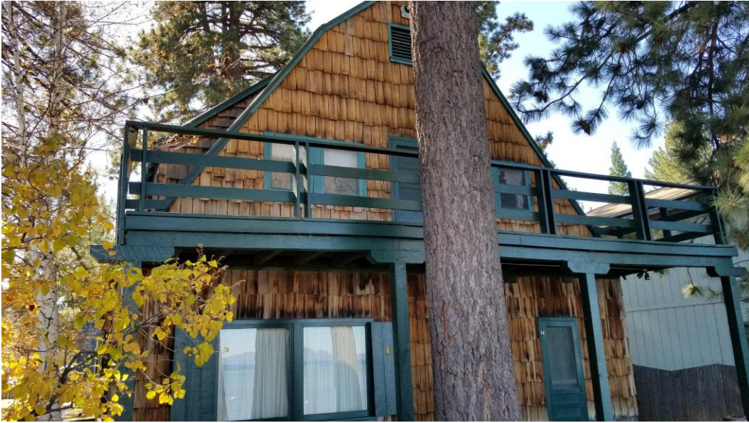
Figure 12. North Elevation of Cabin (Looking south)
