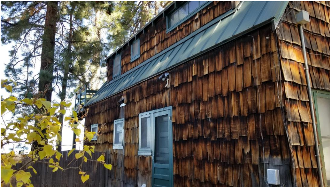
Figure 13. Southwest Corner of Cabin (Looking northeast)
