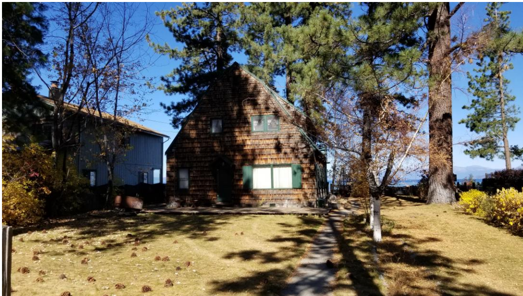
Figure 7. Overview of Cabin (Looking north toward front facade)
