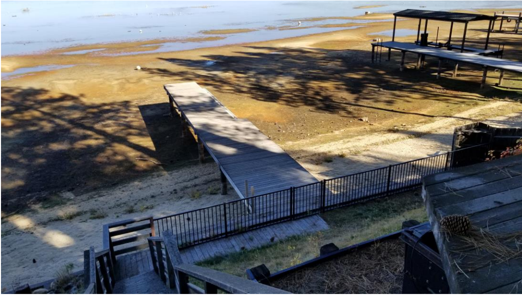
Figure 16. Overview of Pier (Looking north)
