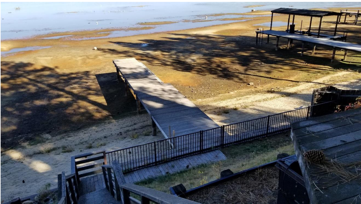
Overview of Pier (looking north). Photograph 103542, E. Johnson, October 20, 2022
