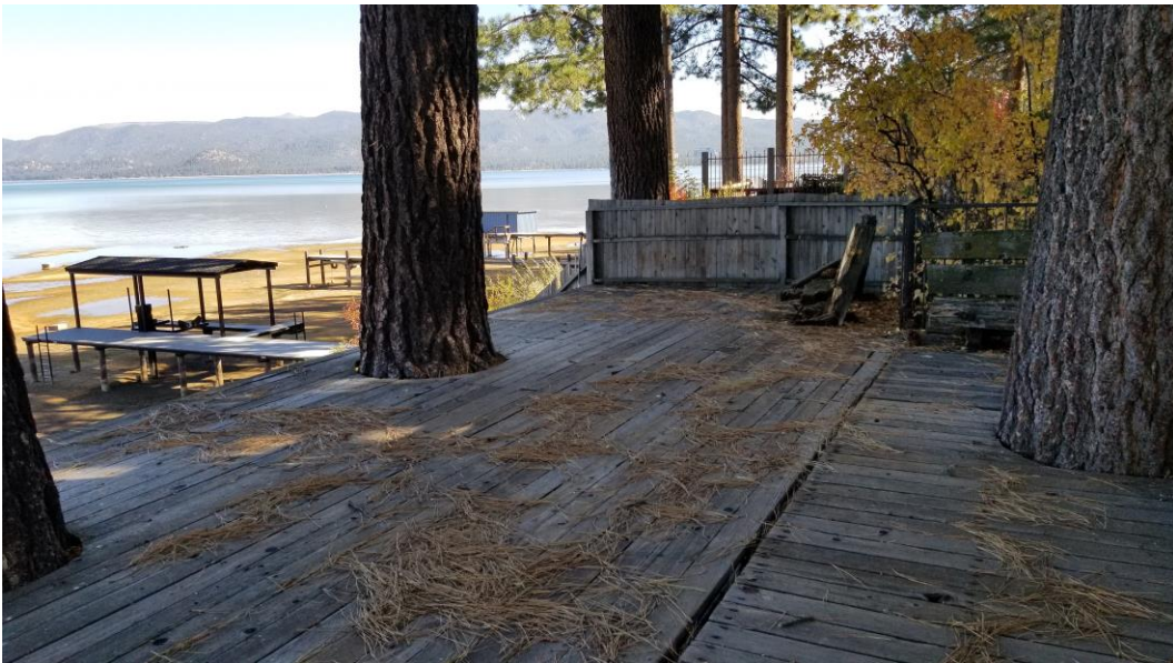
Figure 15. Back Deck (Looking east)
