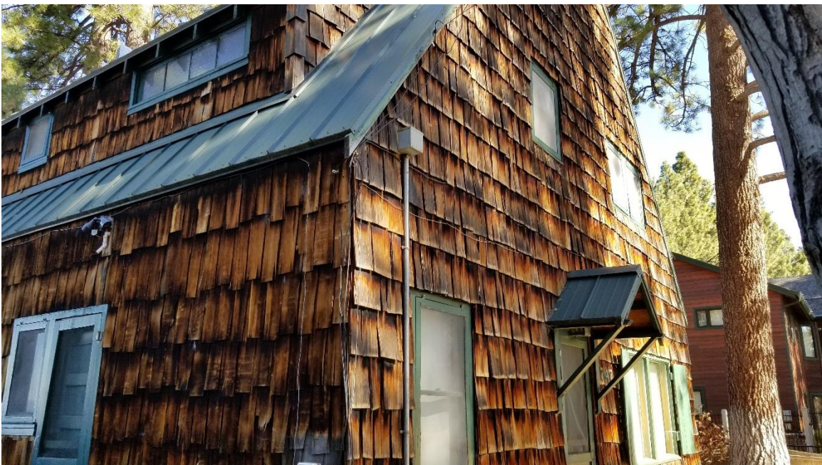
Overview of Southwest Corner (looking northeast). Photograph 120558, E. Johnson, October 20, 2022
