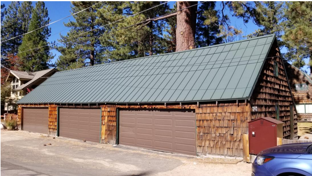
Figure 17. Overview of Garage (Looking northwest)
