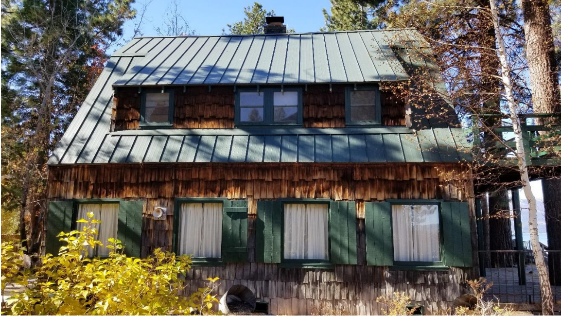
Overview of East Elevation (looking west). Photograph 120237, E. Johnson, October 20, 2022
