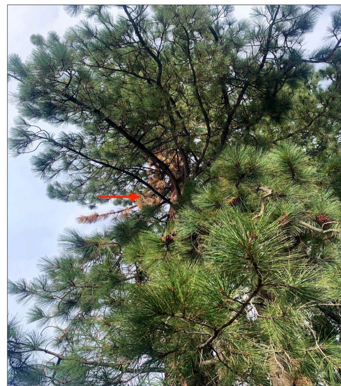
Photo above: red arrow indicates a dead, broken branch hanging in the crown of tree #181, remove to prevent possible injury below.
