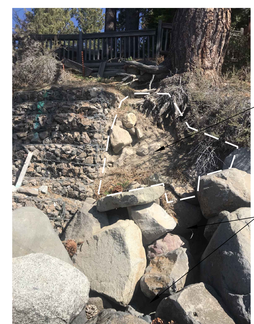
PHOTO OF GABION & BOULDER REVETMENT AT EAST PROPERTY AREA
