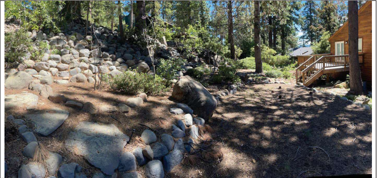
Photo 3 – View to east at upper (north) part of property. The backyard has several created terraces separated by rock retaining walls. At upper left, rock armored surface atop 40 to 55% slopes that were over-steepened when adjacent Dardanelles Avenue was constructed (circa 1970). For land capability matters, TRPA utilizes natural (historic) slopes, which are estimated at 20% for this vicinity.
