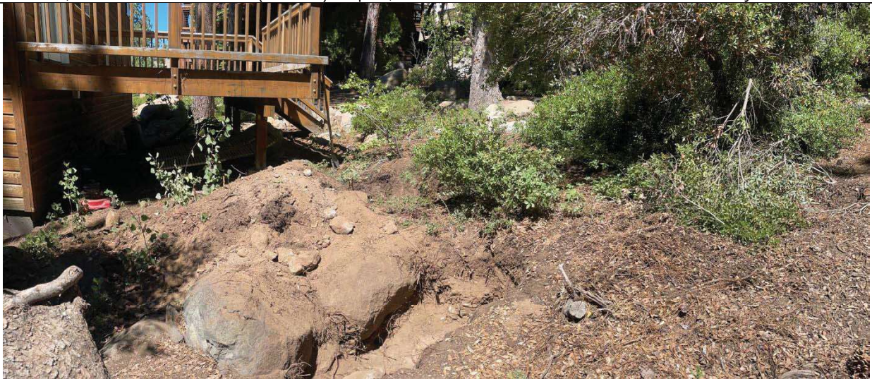
Photo 4 – View to east edge of parcel where sample site 7/25/23-1 was hand-excavated about 15 feet northeast of residence (just east of small deck, behind dirt pile). Slopes are 20% in this vicinity. The test pit showed the property has deep soils that become increasingly rocky with depth.
