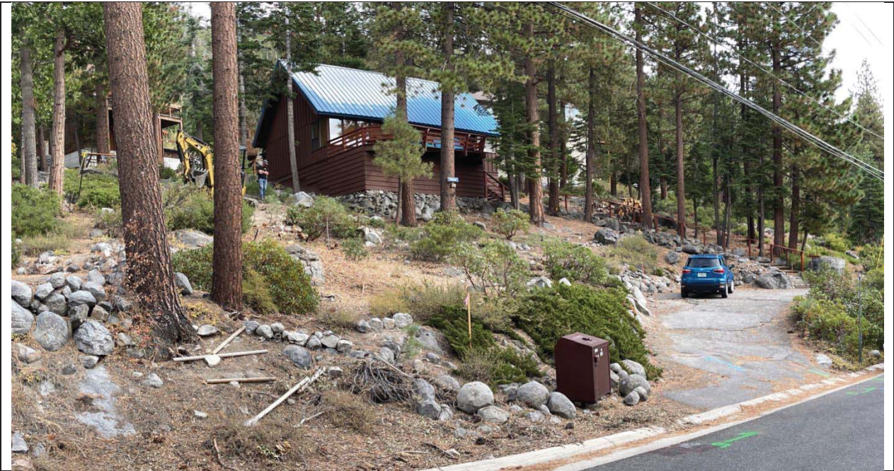
Photo 1 – View to east and southeast from northwest corner of project area. Slopes are 30 to 33% just below the residence. Slopes are artificially steeper adjacent to driveway; however, historic slope condition is utilized for land capability challenges.
