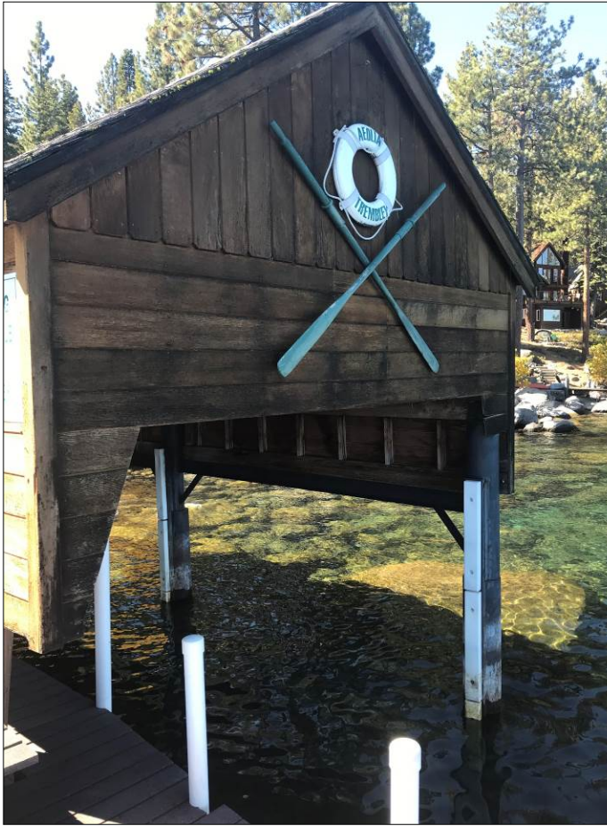
Boathouse, view northwest, lakeside. IMG-6250, 10/17/2020.
