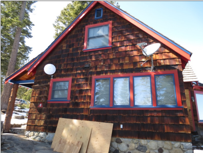
Primary Residence, view northwest, 3/7/2021
