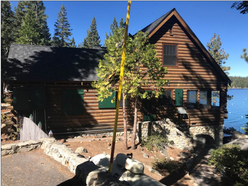
Southeast Elevation of Primary Residence, 10/17/2020
