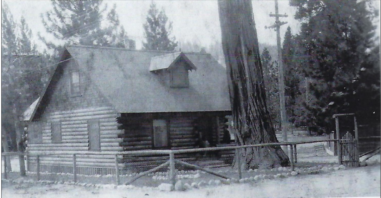
Figure 7. Caretaker's Cottage at Meeks Bay Resort, 1931.
