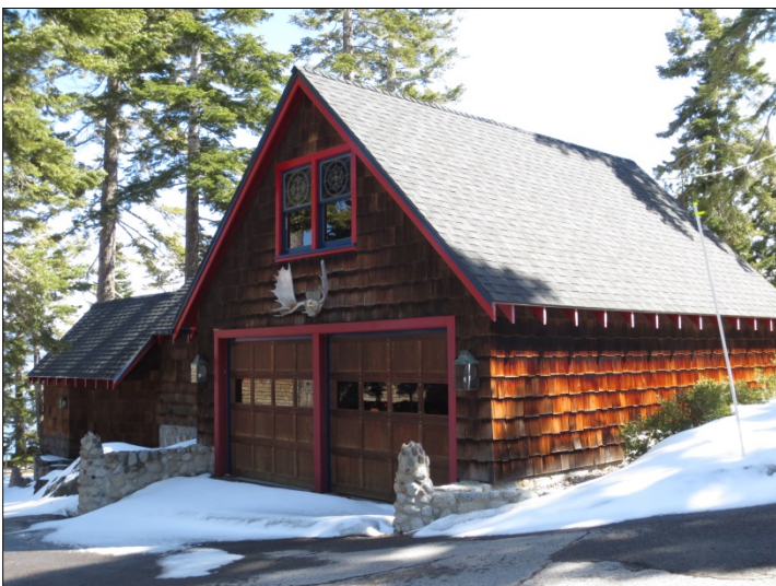
Garage and Guest House, view southeast, 3/7/2021
