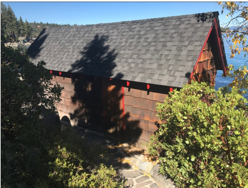
Pump House, view northeast, 10/17/20, IMG-6170 (above); mortared stone foundation (right), IMG-6245
