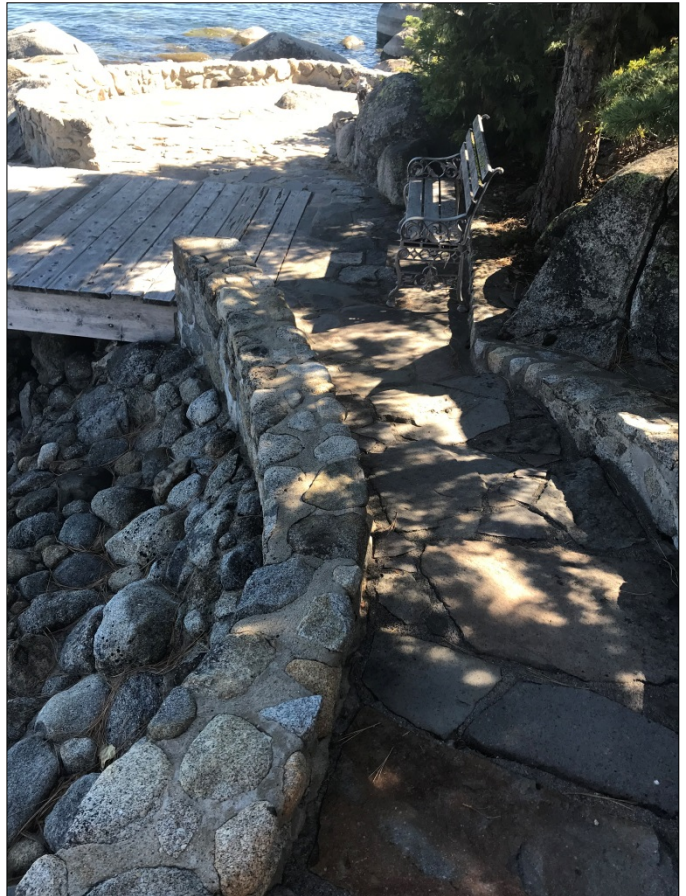
Mortared slate and stone path to mortared stone landing, lakeshore, 10/17/2020, IMG-6138
