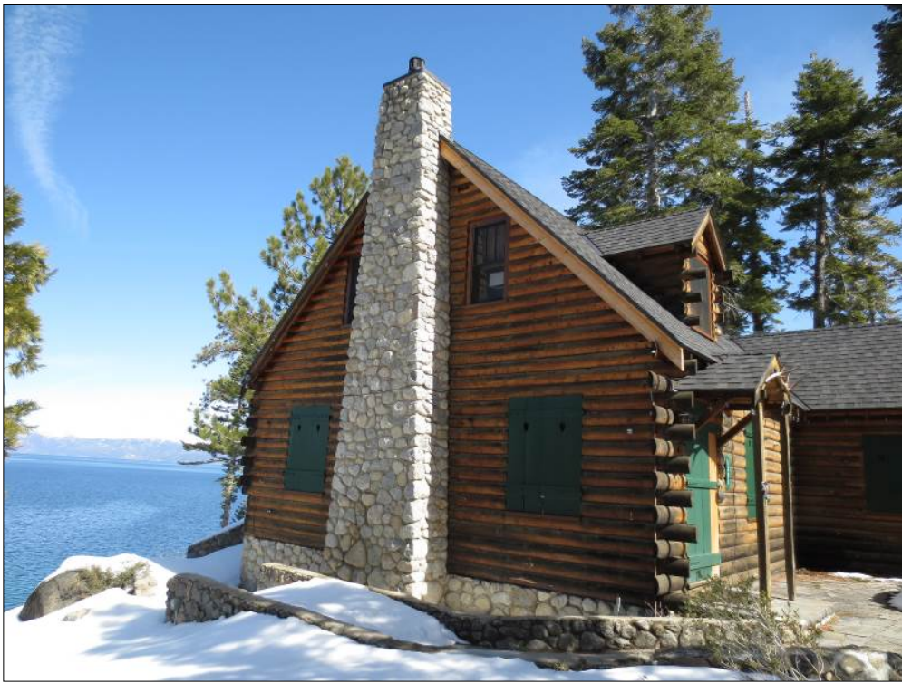
East Side of Primary Residence, view east, 3/7/2021
