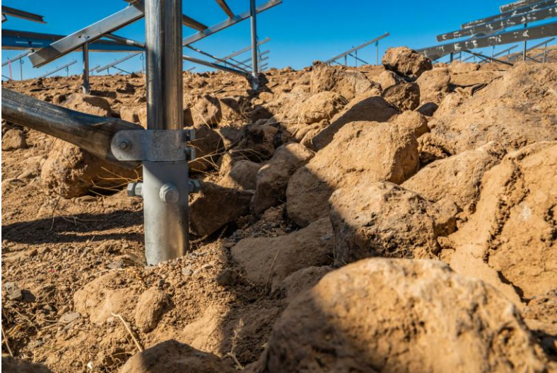
Example of solar array structure using ground screws
