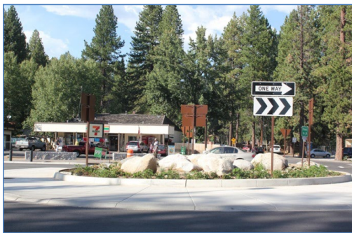
New roundabout in Kings Beach
