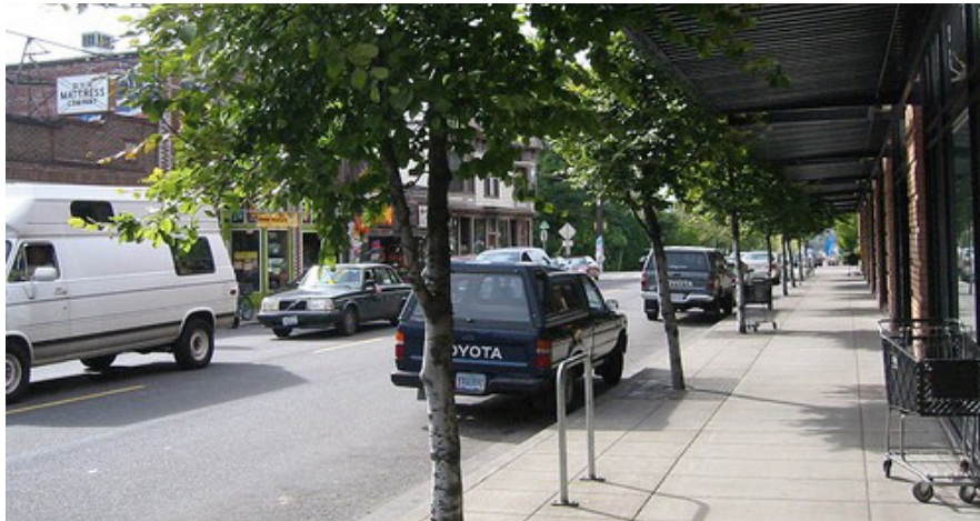
Concrete Surfacing (non local)
