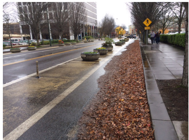
Fallen leaves accumulating separated bike lanes cause hazardous conditions in wet weather.
