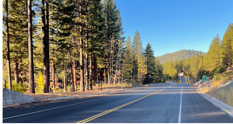
Church Entrance From Mt. Rose Hwy
