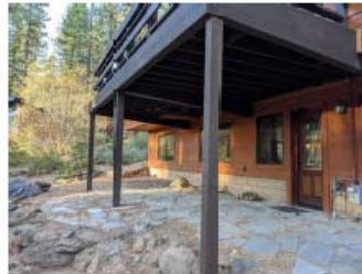
Figure 2 Overview of temporary deck posts, existing patio
