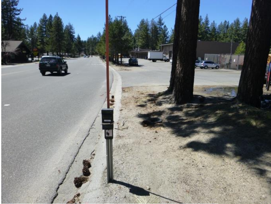
A monitor located on Al Tahoe before the Al Tahoe Safety and Mobility Project
