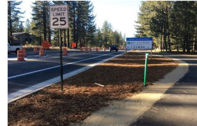
Post Construction - Al Tahoe Blvd WB New Class 1 Path
