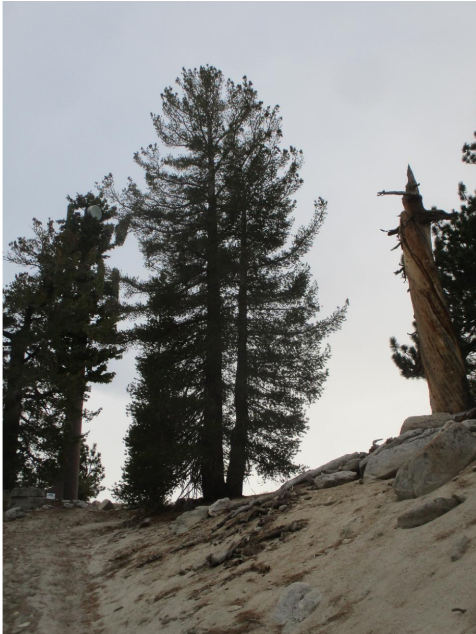
Angel's Roost tower approach road, very steep, erodible. Native tree at center. Faux-pine tower at left. Needles were replaced in 2022.
