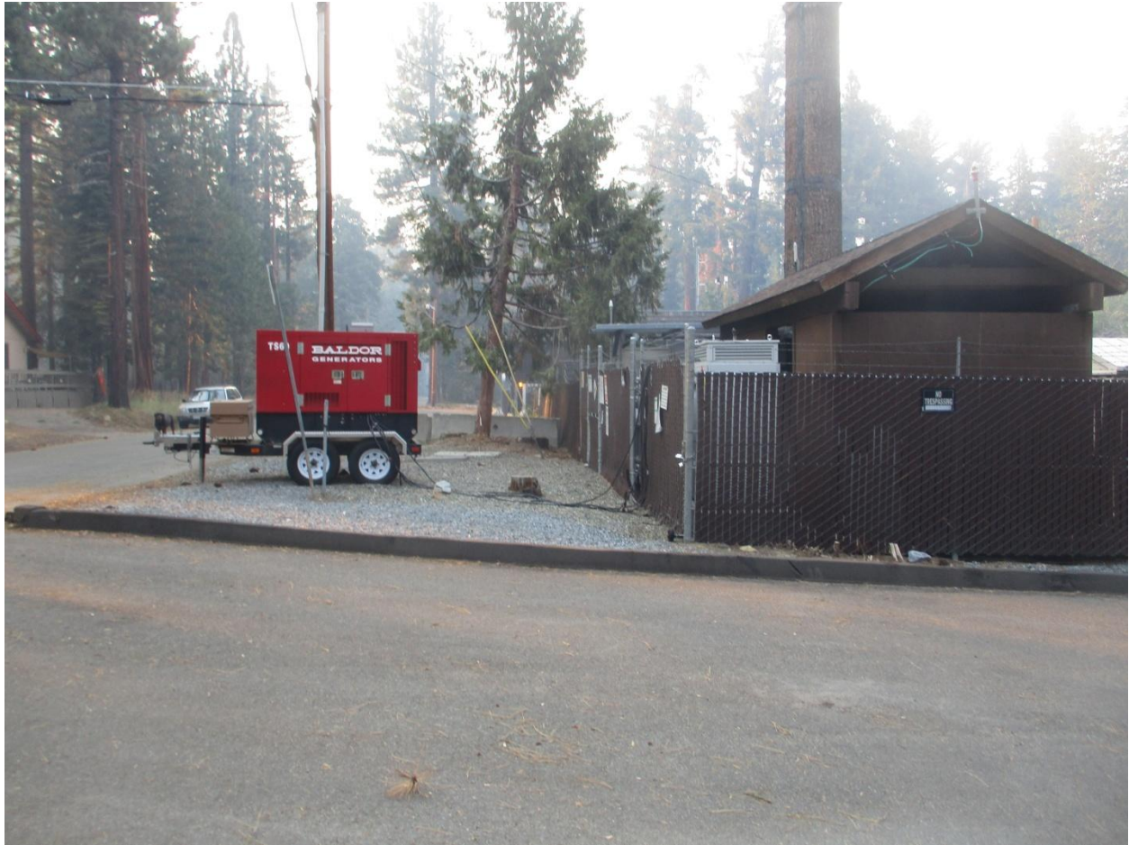
Wilson Ave tower site, Wilson Ave at left, base station, trunk at right, near roadway. Portable generator parked in right of way, off the Project site. Drainage flows are towards viewer. Fallen needles/fragments are difficult or impossible to remove from gravels (grinding stones).
