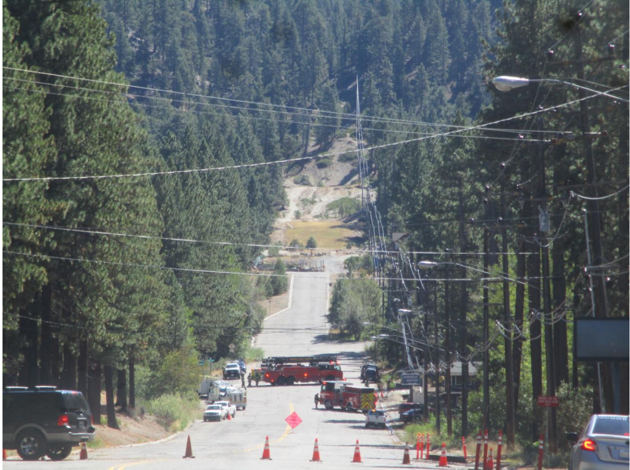
Needle Peak and Ski Run Blvd. closed, neighborhood evacuation for gas line break by Verizon contractor. 9/22/22
