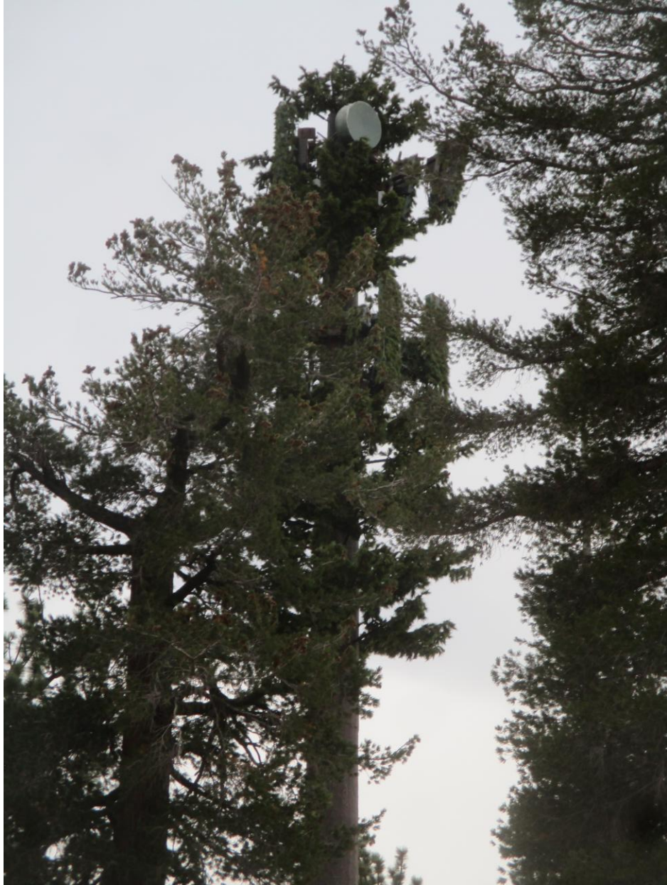
Angel's Roost tower. Note tree top sheared off in foreground.
