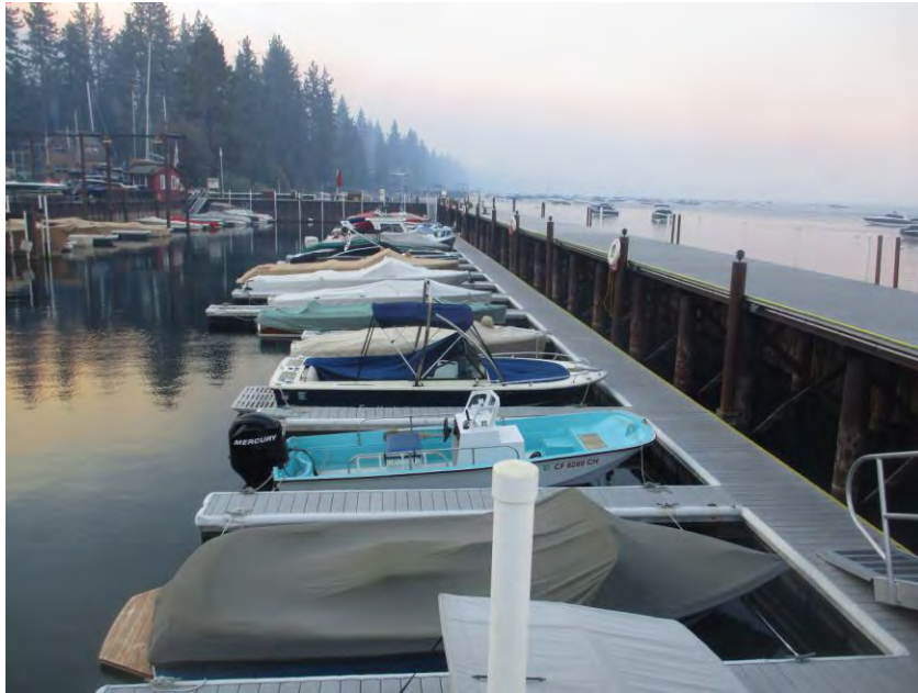
Looking northerly, fuel dock on far end. (5449)
