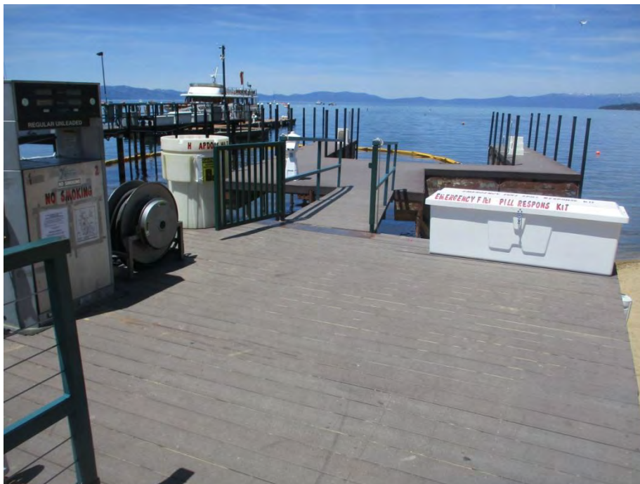
Ski Run Marina, looking north. Lots of plastics, generally in reasonably good condition, though still subject to abrasion by sand, as shown in cracks, and weathering. Note turbidity curtain surrounding (yellow). (4234)
