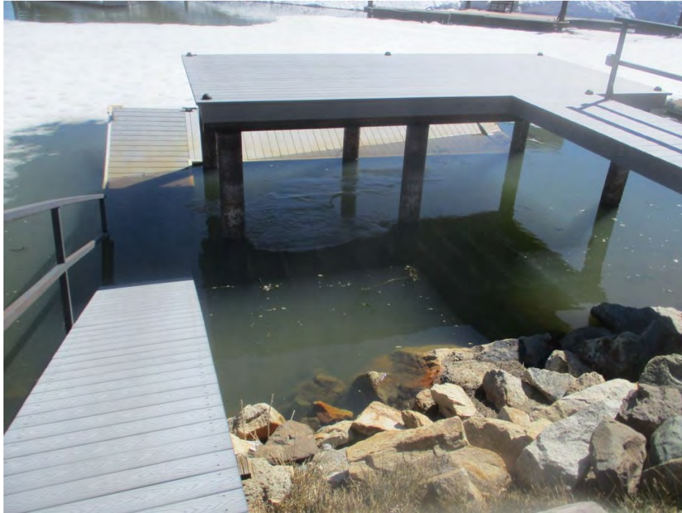
Submerged plastic dock, typical of the many that will require repairs following the winter of 2022-2023. (7513)
