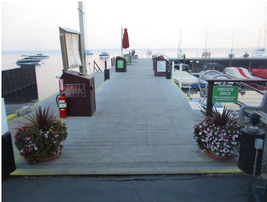
Looking easterly, fuel dock on far end. Note severely degraded plastic decking at entryway. All of the observed decking is in a state of decay at this marina, while still capable of serving functionally. Observations at Obexer’s marina include a high number of degraded deck boards, plastic with breakage, cuts, chips, abrasion and general deterioration, as follows. (5454)
