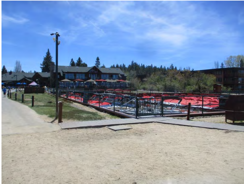
Ski Run Marina, with its rental boat fleet, looking south, with plastic decking laid on sand near beach, abraded by sandy shoes, walkers, equipment. (4229)
