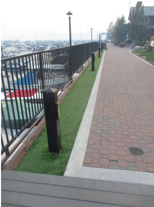
Plastic astroturf along entire length of sheet piles. (5476)
