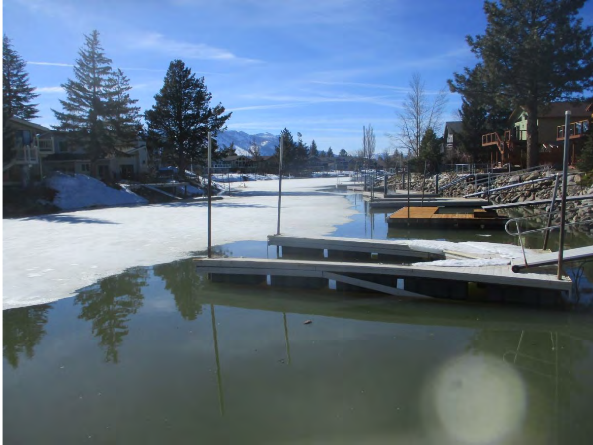
Note the number of submerged, damaged docks, especially on the far bank. 8/20/23 (7643)
