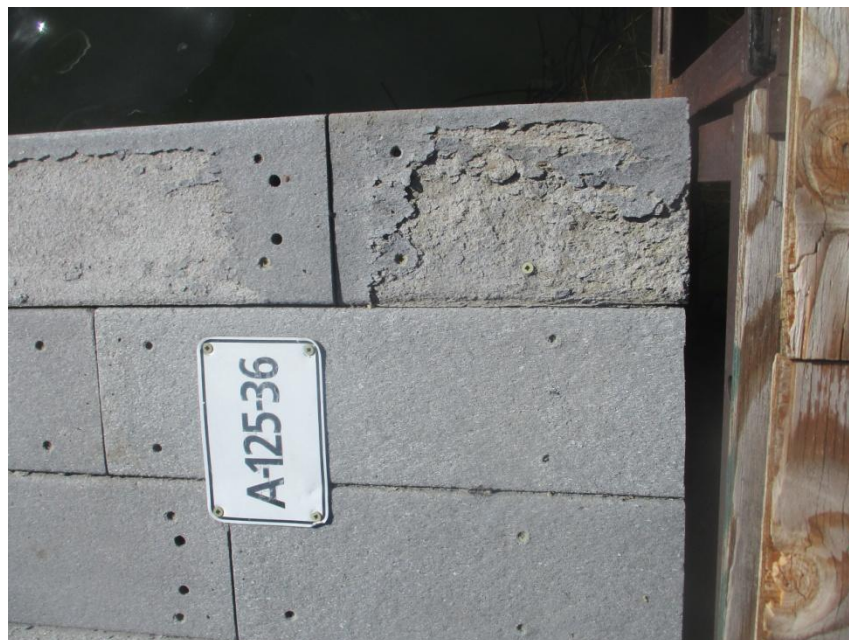
Plastic decking deteriorated from weathering and flaking off as microplastics over waters. Typical of the hundred of plastics docks at Tahoe Keys Marina. (7982)
