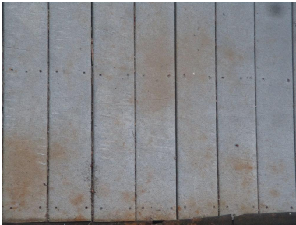
Weathered, scuffed, scratched, stained decking. (5485)
