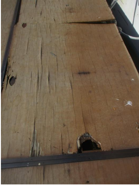
Deteriorating weathered plywood. (7993)
