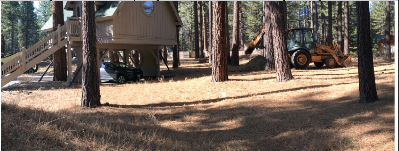
Photo 3. View southwest to west (right) at Soil Pit 1. Carport/office at left. This portion of the parcel has a thin veneer of fill material, 2 to 6 inches thick (presumably placed during prior construction).
