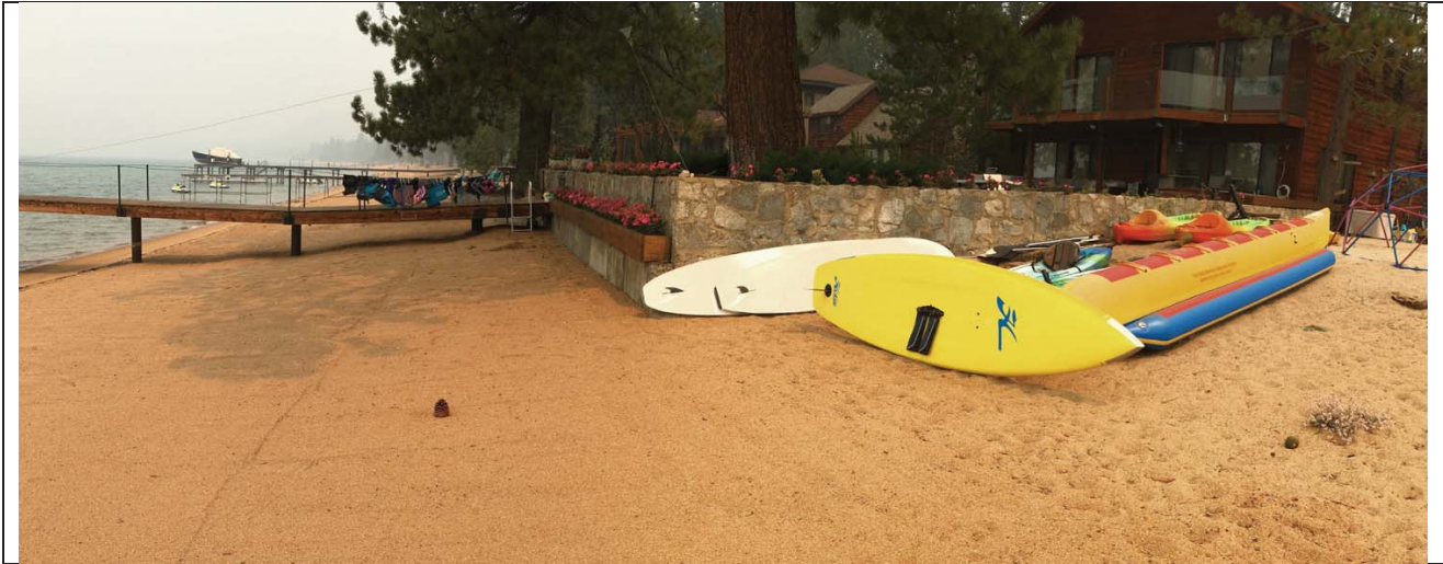
Photo 3 – View north toward southwest property corner. Subject residence located at far right and Lake Tahoe at far left. The retaining wall was built (and likely rebuilt) to prevent further erosion of the shoreline and protect several large Jeffrey pines. Without the retaining wall, the land on the adjacent parcel (foreground, right) has eroded away a portion of the stabilized barrier beach ridge.
