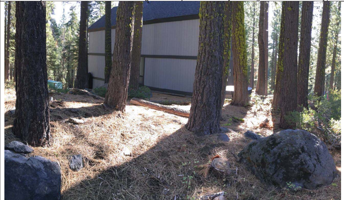
Photo 4 – View to northeast of southwest property corner (highest elevation). This vicinity has several very large boulders. These are not anchored to bedrock, which is deeper than 6 feet below the surface. Slope is roughly 18% to the northeast (left) and east (right).
