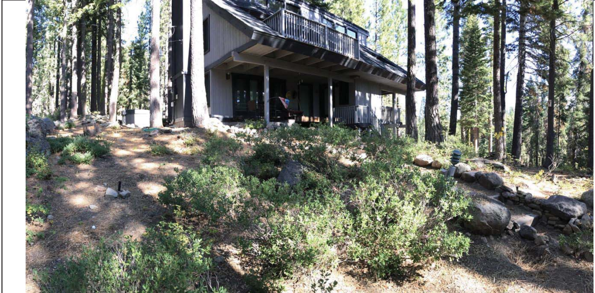
Photo 1 – View to northwest from southeast portion of property. Slopes are 24% in the left half of photograph and 15% in the right half (E and NE aspect). Sierra Vista Avenue located in opposite direction (behind photographer). Immediate foreground is artificially steepened by driveway cut.
