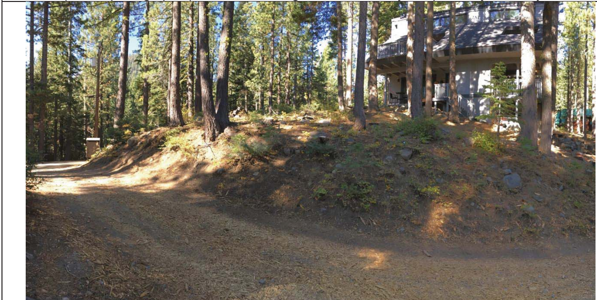
Photo 2 – View to south at southeast edge of parcel where driveway was excavated across the hillside to allow access to the residence from a less steep slope. For land capability challenges, TRPA utilizes the historical slopes, so these excavated slopes are designated as Class 4 (instead of Class 2 for slopes greater than 30%).
