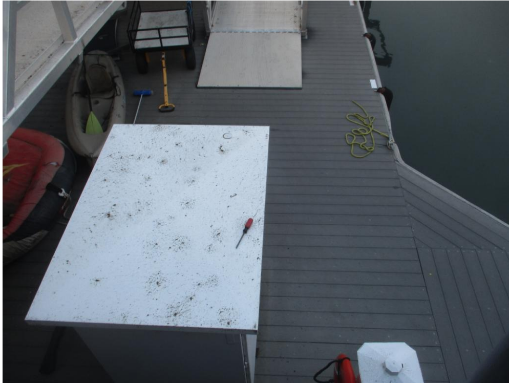
Example of decking in the older sections, ramp at top of photo. (5464)
