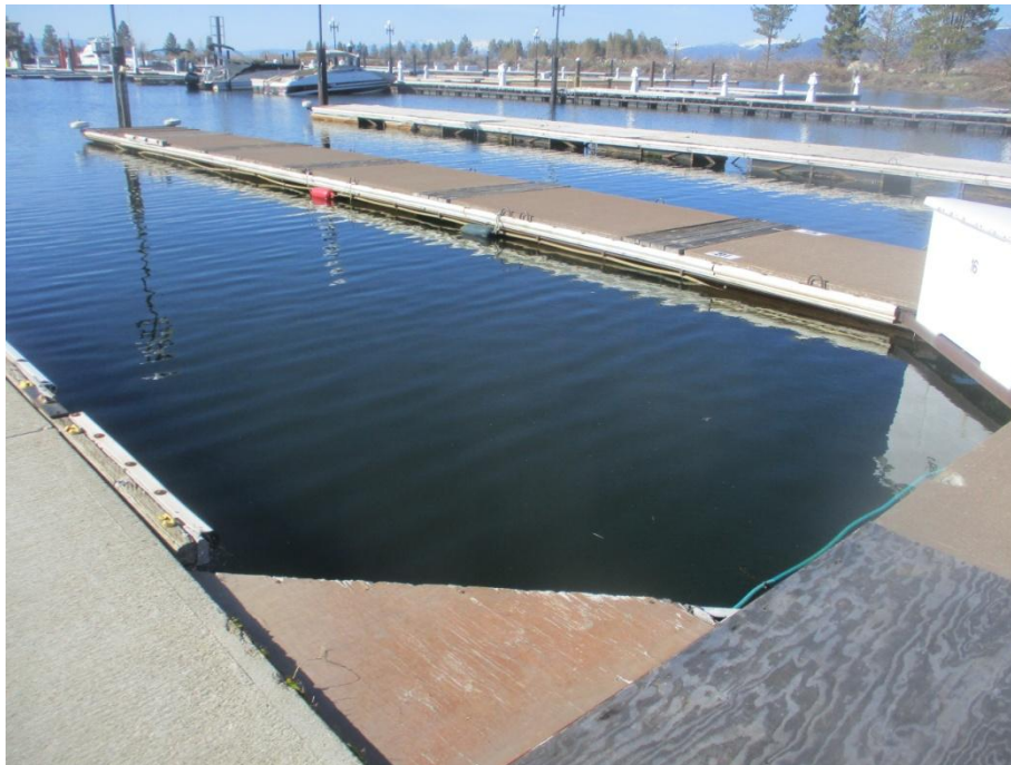
Some older pier decks are concrete, which hold up better, or wood. Here is a floating dock extension (above center pier, whitish) that is partly covered by plastic sheathing. (8011)
