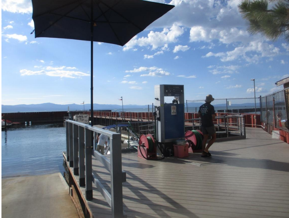
Small marina. Wrap-around plastic decking, generally in good condition, adjacent boat ramp. (50 31)
