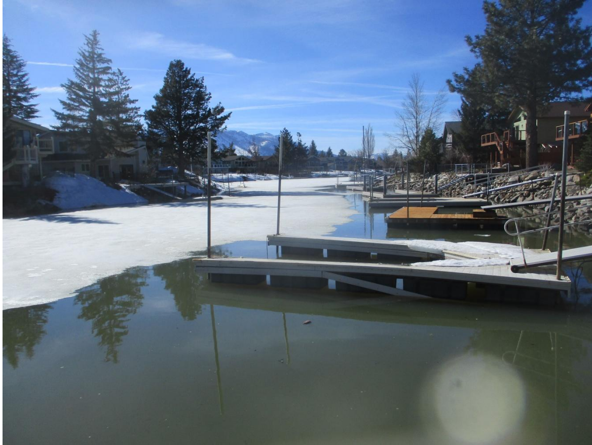
Note the number of submerged, damaged docks, especially on the far bank. 8/20/23 (7643)
