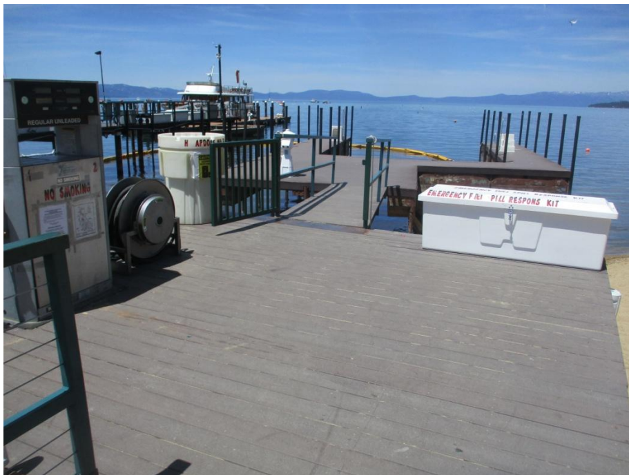
Ski Run Marina, looking north. Lots of plastics, generally in reasonably good condition, though still subject to abrasion by sand, as shown in cracks, and weathering. Note turbidity curtain surrounding (yellow). (4234)
