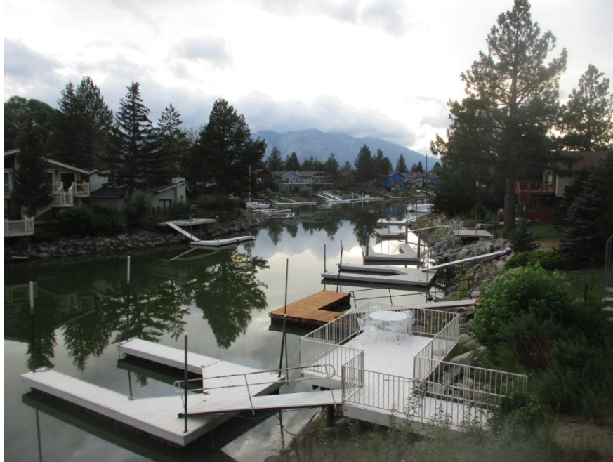
Tahoe Keys Lagoon, west of Lido, 8/5/22, after dual treatments for AIS. Note intact docks and piers, algal bloom, poor water quality, waters closed to boating (“the lost season” for many). (5003)
