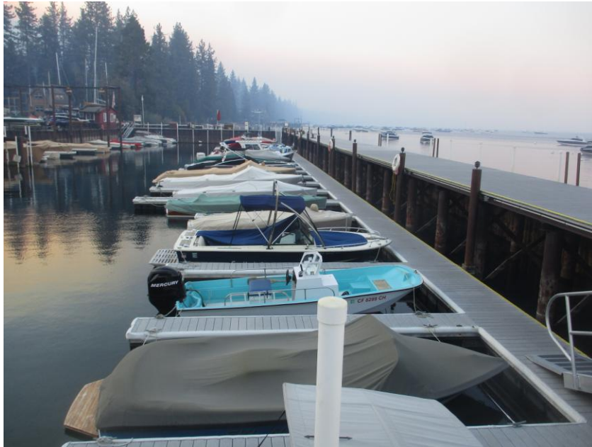
Looking northerly, fuel dock on far end. (5449)
