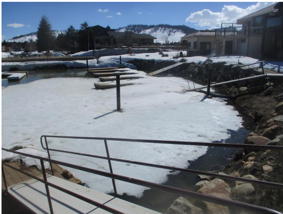
Plastic docks buried and broken by winter snow and ice, Spring 2023. (7519)
