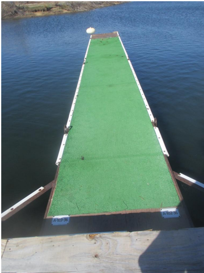
Plastic carpet over plywood. Such plastic turf replacements are not uncommon at the marinas I visited. Green color, attractive to waterfowl. (7991)
