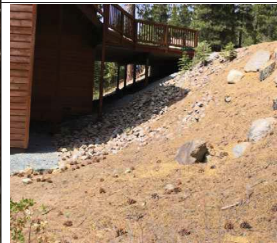
Photo 7 – View north at steep embankment between residence and Eagle Drive. The steep, fill slope was created by original road construction and now has ground cover as scattered shrubs and pine needles/twigs. For land capability purposes, TRPA acknowledges the historic slope, which is estimated as 23 to 29% (steeper toward south prop. line.). Class 4 has a slope range of 16 to 30%.
