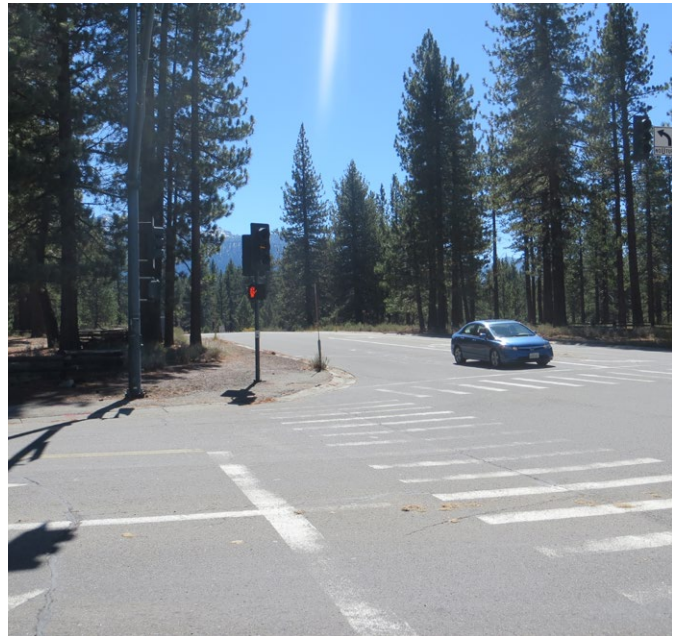
Lack of curb ramps at the Al Tahoe/Johnson intersection
