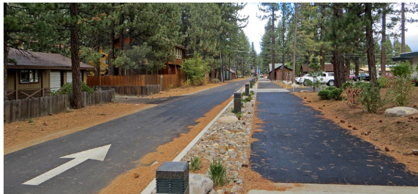
Example of Class I separated bike path
