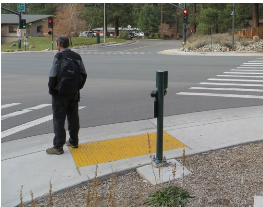
Example of flared curb ramp
