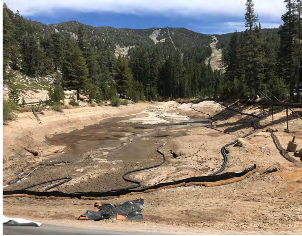
Prior to Dredging in Early August, Diversion all set up.
