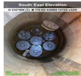
New filters installed
