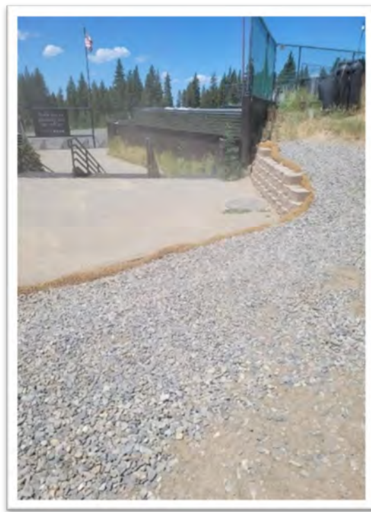
After: Drain rock buffer installed behind the Lodge between access and patio.
