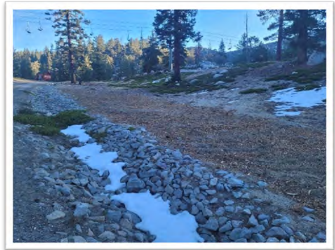
After: "Rip and chip" treatment on shoulder and refurbished rock-lined swale.
