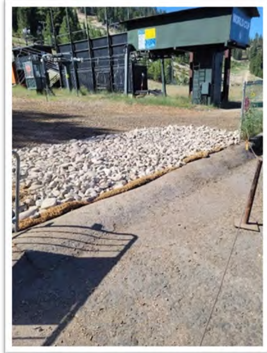
After: Rock riprap buffer at parking lot entrance.
