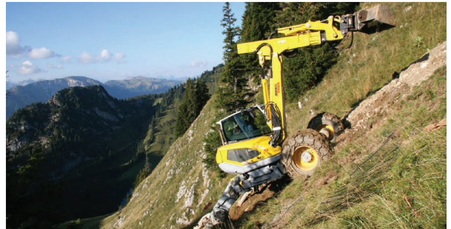
Figure 4.40: Spider excavator on steep slope (photo by www.dozr.com )
