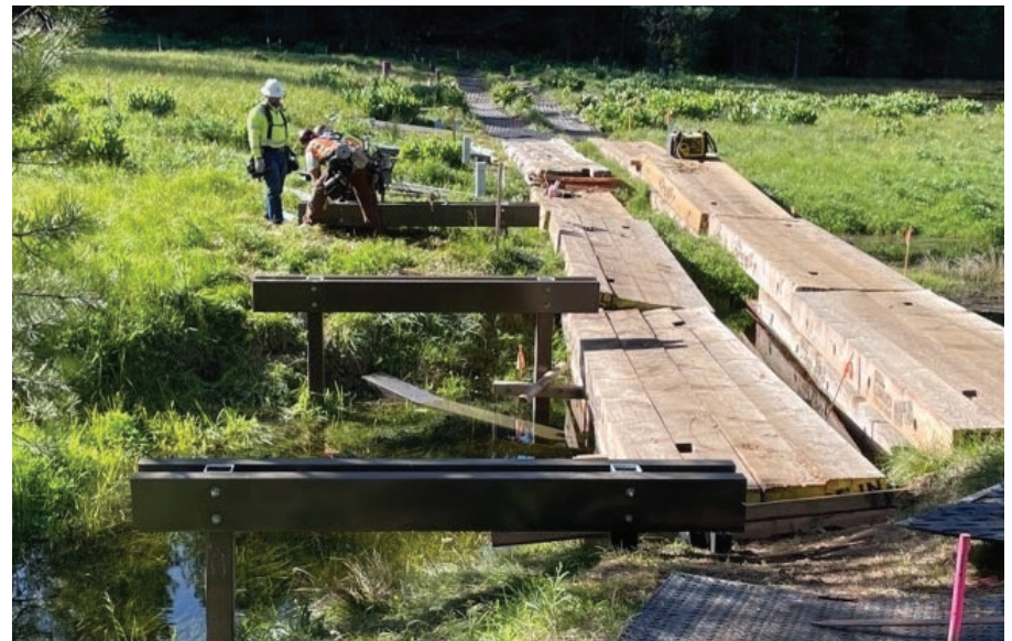
Figure 4.23: Micropyle installation for boardwalk through sensitive riparian habitat (photo by P. Preston).
