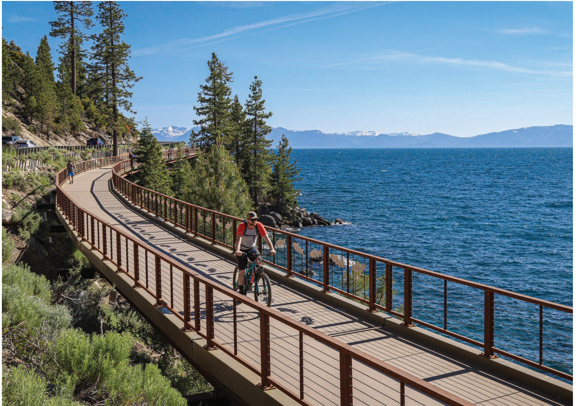
Bridge along Tahoe East Shore Trail (photo by Shaun Hunter from outdoorproject.com)
