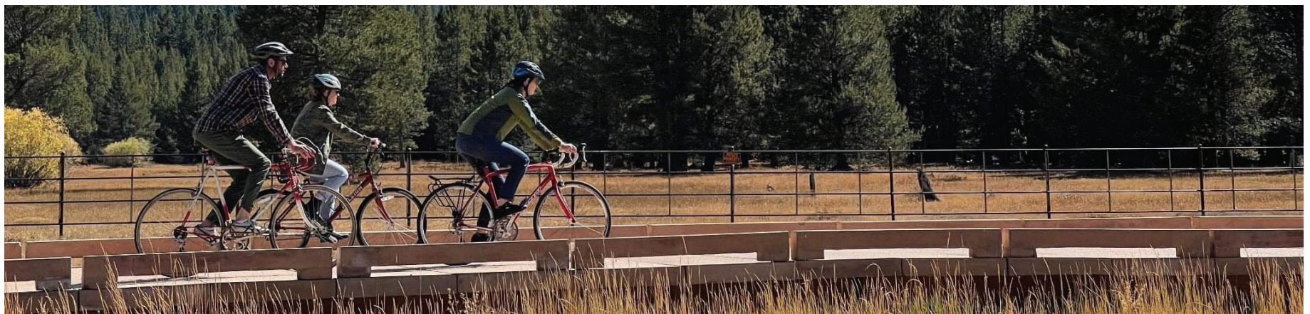
Figure 3.20: Example of boardwalk through a stream environment zone in South Lake Tahoe (Photo by C. Carney)
