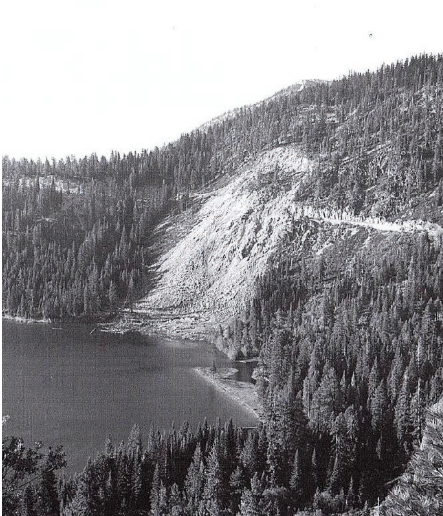
Figure 3.16: Emerald Bay landslide circa 1956 (photo by S. Gennerich)
