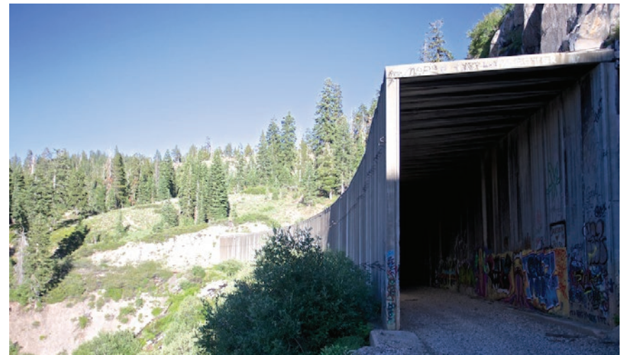
Figure 3.18: Tunnel along abandoned railroad above Donner Lake, California (photo by Josh McNair from Californiathroughmylens.com )
