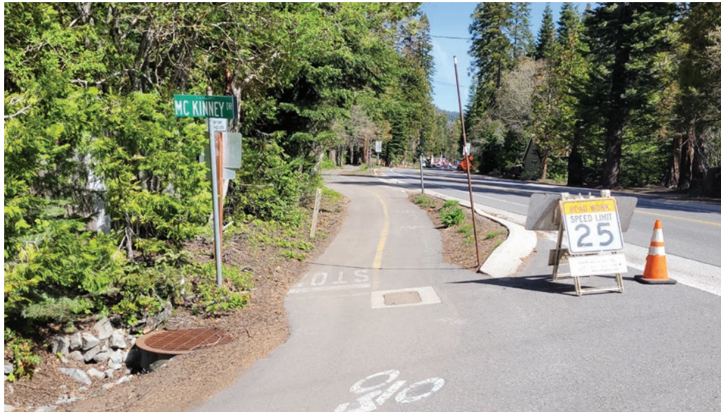
At-grade screened bike trail along west shore of Lake Tahoe (photo by D. Rios)
