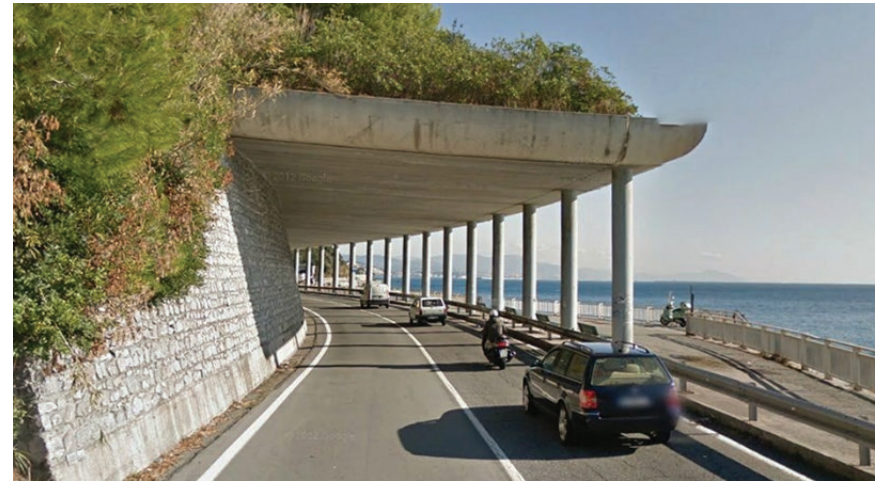
Figure 3.17: Flat rockshed example (photo by www.larimit.com )
