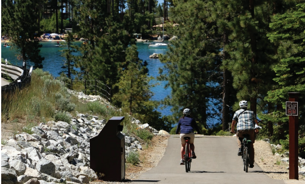
Tahoe East Shore Trail on steep slope (photo by Jason Bean from Reno Gazette Journal)
