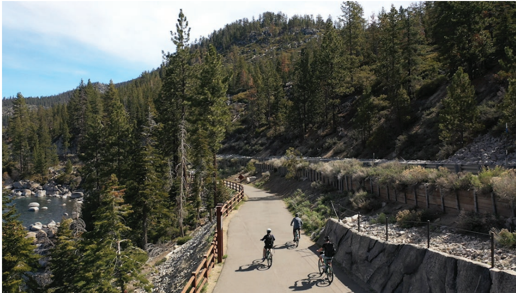
Tahoe East Shore Trail on steep slope (photo by nevadasportsnet.com)
