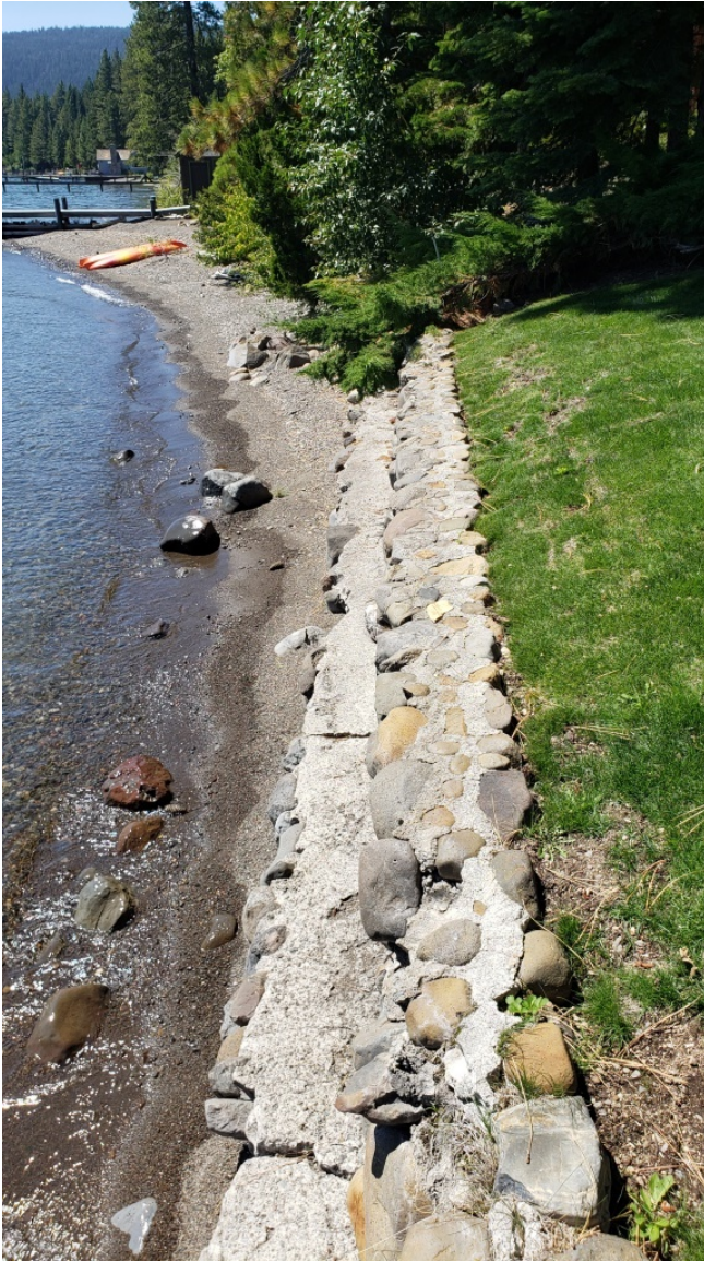
Easterly view of existing retaining wall, 2020
