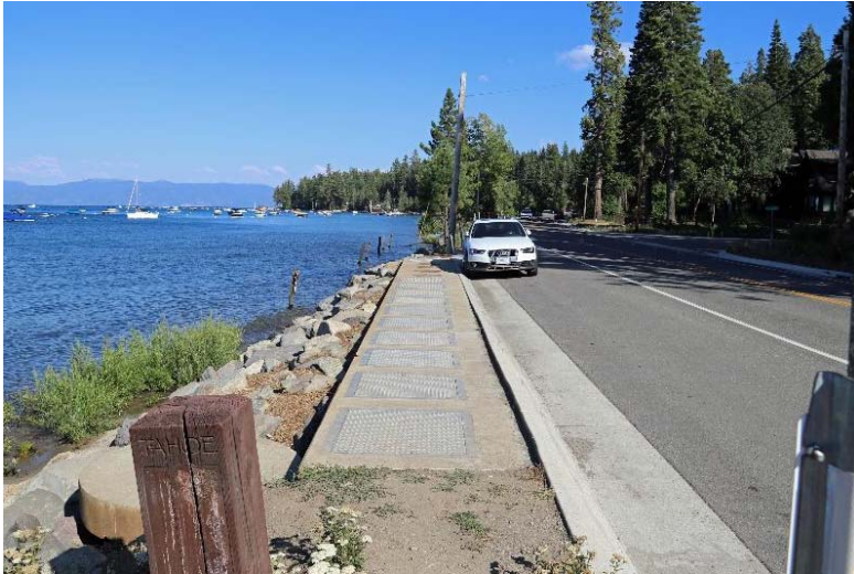
Sand vault treating stormwater before it discharges to Lake Tahoe, constructed as part of the State Route 89 water quality improvement project. (Photo credit: Caltrans)
