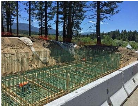
Installation of a Delaware sand filter near the Upper Truckee River in July 2018 as a part of the U.S. Highway 50 "Y" to Trout Creek project (Credit: Caltrans)
