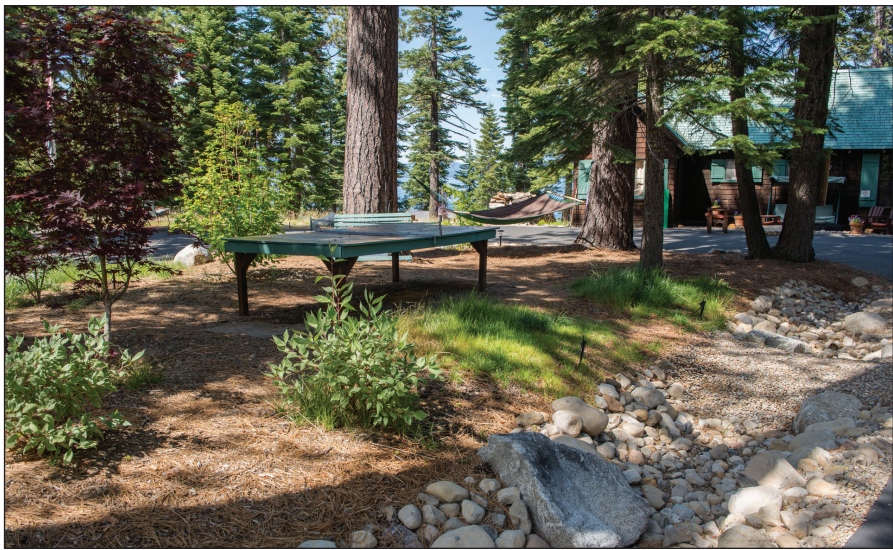
The owners of this Tahoma home installed rock-lined bio swales to treat stormwater runoff.
