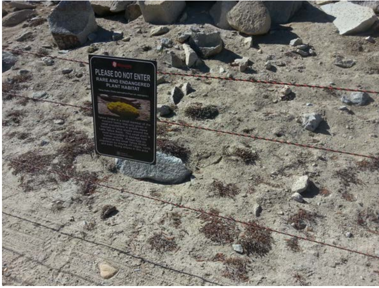
Photo N – Resource Protection Fencing example. Three rope minimum, stakes to be placed at a maximum distance of 20 feet.
