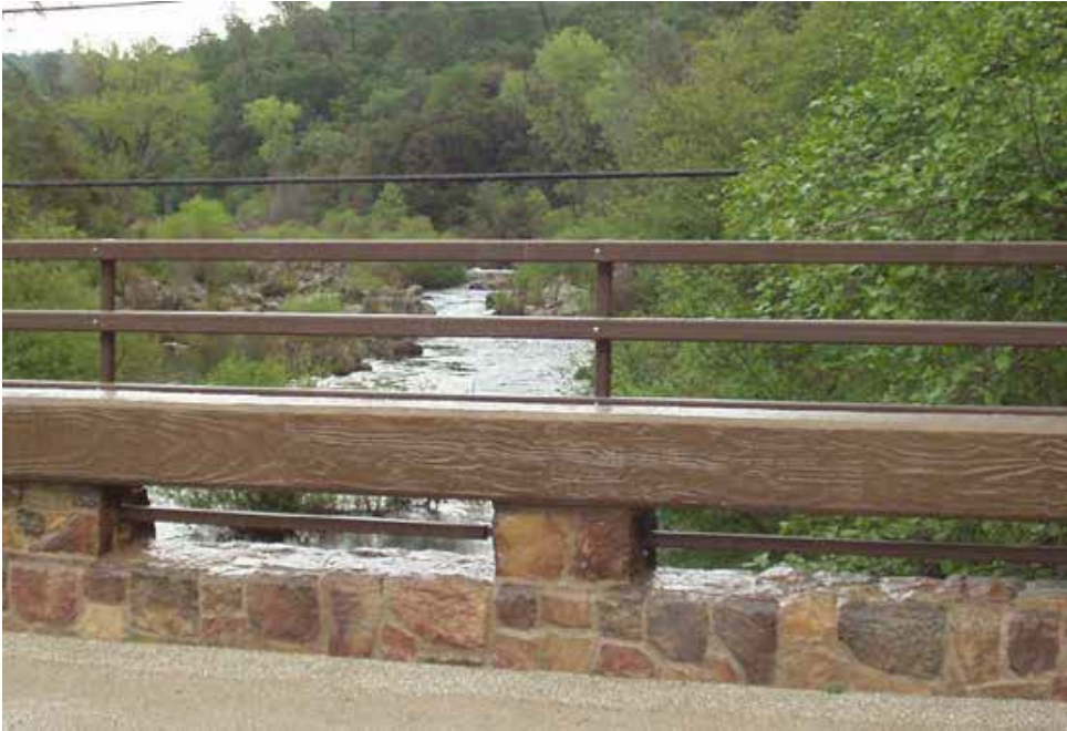
Vehicle Barrier: Concrete barrier with wood like texture
