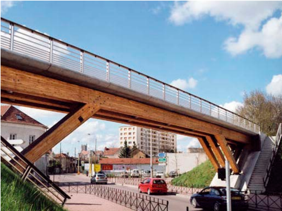
Pedestrian Bridge: Glued laminated timber with exposed architectural hardware
