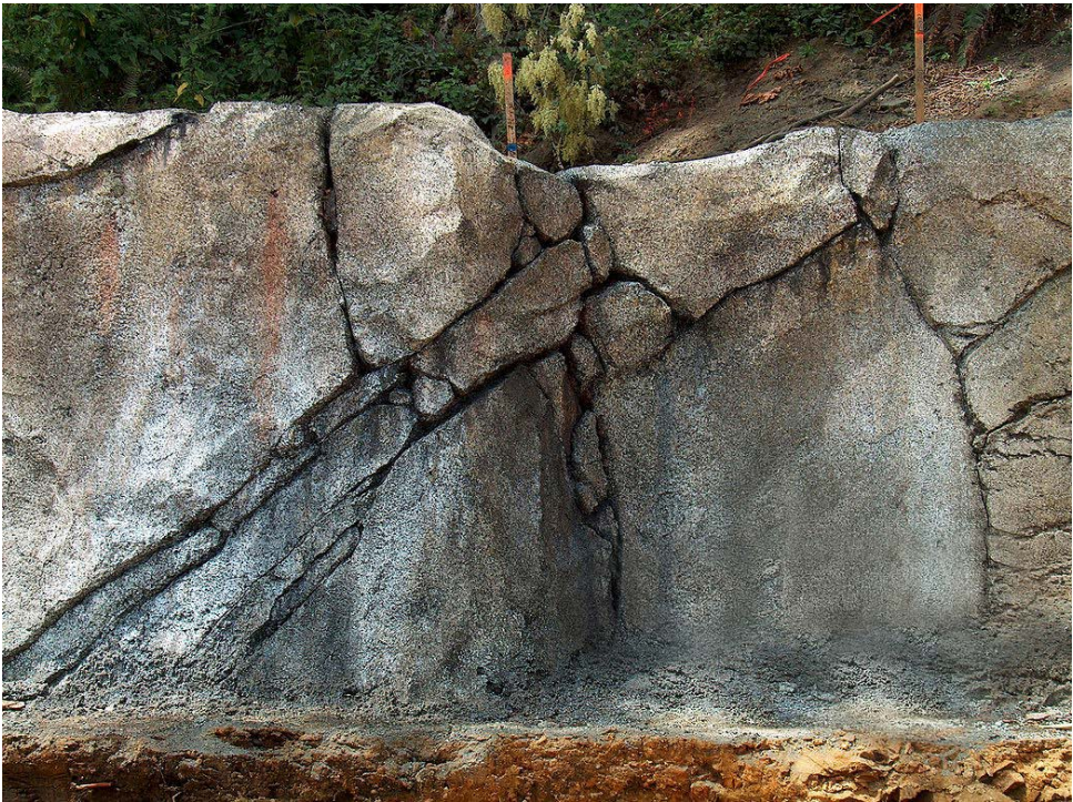
Bridge Feature Wall: Customized sculpted concrete to mimic natural granite outcroppings
