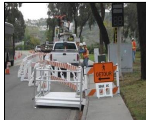
Example where pedestrian detour is clearly marked, has detectable delineation, and temporary curb ramps.
