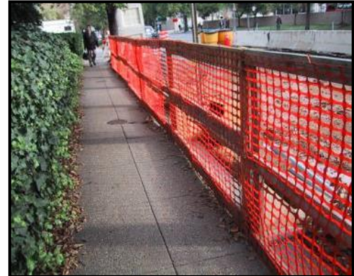
Example of a temporary barrier that may be used across a sidewalk to close it or to separate pedestrians from work area. Including a top rail and base rail to be detectable.
