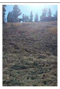
Infiltration area added upslope to address source of runoff; Full Hogan treatment on slope. PROBLEM IDENTIFIED AND TREATED IN SAME SEASON!
