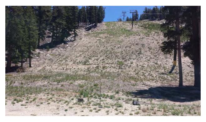
Double Down Lower after Full Restoration Treatment. 2 full run width Pine Needle Filter Berms above Infitration/Vegetated Swale.
