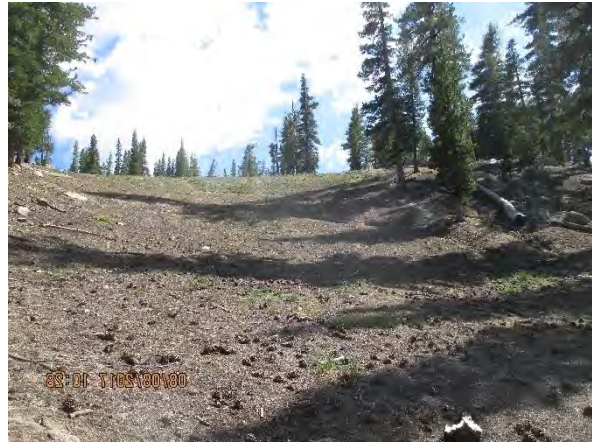
After: Infiltration spreading area created by loosening deep gully and restoring it as in an infiltration swale.
