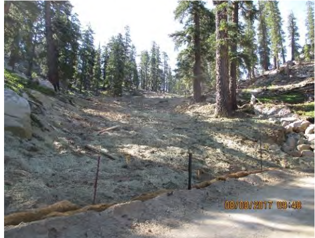
After: Area hydroseeded, tilled and mulched. Riprap channel directing flows to culvert under road.
