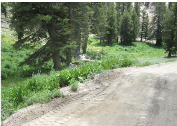
Before: very steep section of road (Hellwinkel's) delivering sediment downslope near SEZ channel above Sky Meadows culvert. Rills and gullies formed on hillside below road and above channel.
