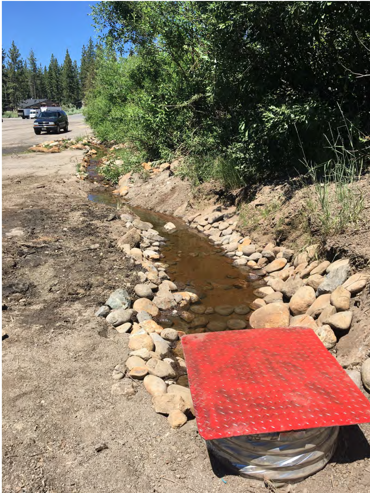
French Drain improvements and a blind vertical culvert inlet installed at California Lower Parking lot July 2017:
