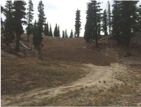
Before: Sediment plume and incising waterbars downslope of road, all caused by concentrated road runoff.
