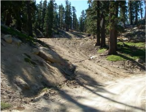
Before: Bare ski slope impacted by drainage from switchback above & drainage flowing across roadway.
