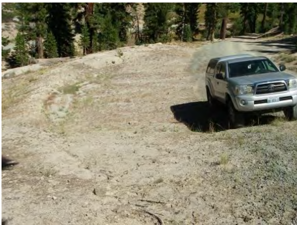
Before: Water bar creating quasi-basin off Maggie's, which overtops to down drain direct to creek when full.
