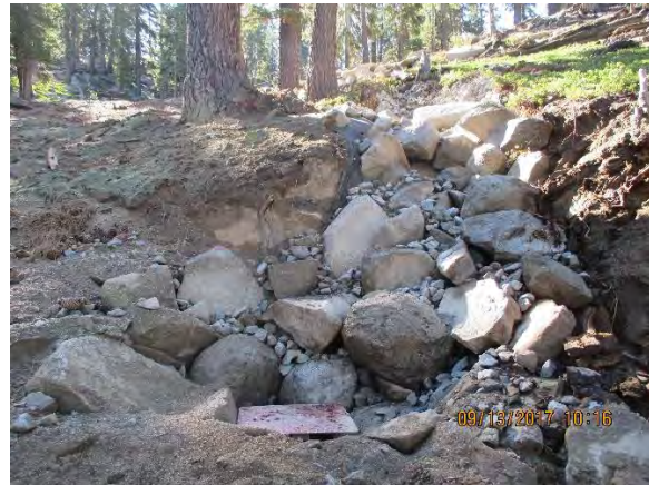
Hand Grenade Chute After: rock riprap protection on gully with geotextile and covered culvert inlet to pass flows across roadway
