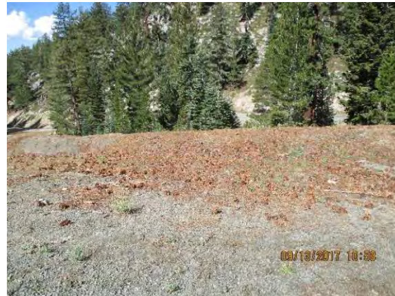
Maggie's Run After: erosion resistance significantly improved with pine needle mulch and regrading of water bar acting as a basin
