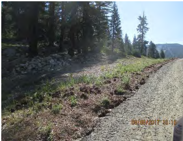
Maggie's Run After: gully formed alongside road improved with pine needle mulch
