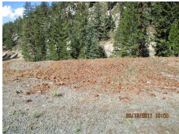
After: Minor reshaping of "basin" area & chip & rip treatment to maximize infiltration and reduce overtopping and runoff to the creek.
