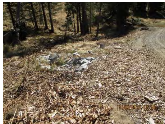
After: Road treated with surface stabilizing agent in 2016. French mattress drain installed to prevent spring from daylighting on road. Both water bar outlets have multiple wattles and rock riprap to protect minimize erosion and sediment transport to meadow/creek. Annual maintenance of treatments.
