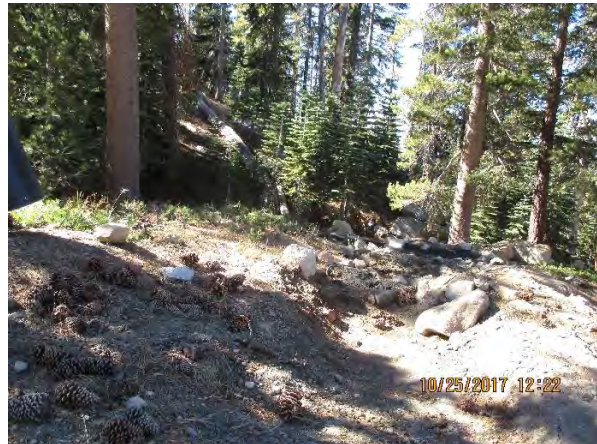
After: Road shoulder ripped and chipped to spread and infiltrate runoff; pine needle wattles added as sediment barrier.
