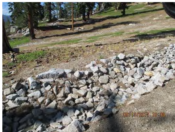
After: Stabilized bare soil areas with full restoration treatment and mulch filter berm. Sediment removed from rock lined channel below sediment plume area.
