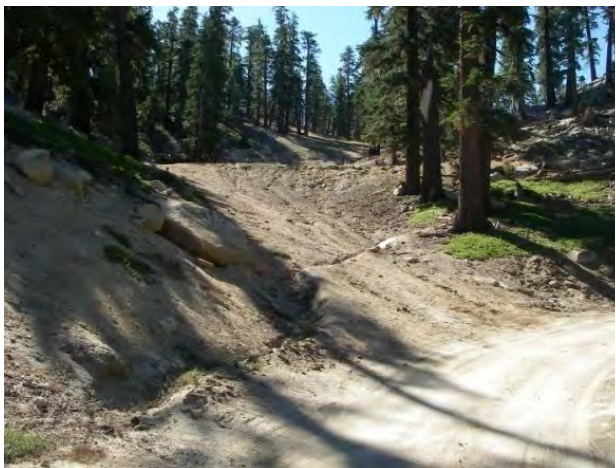
Hand Grenade Chute Before: bare soils, rilling, water bar minimally functioning
