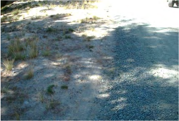
Before: Small gully connecting road runoff to creek.
