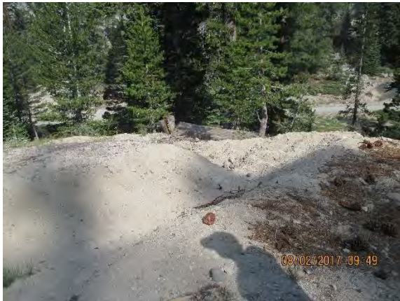
Maggie's Run Before: bare soils, waterbar not functioning properly
