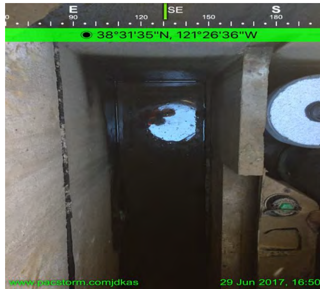
Outlet bay clean and clear of sediment. Repairs to outlet bay holding well. No maintenance recommended.
