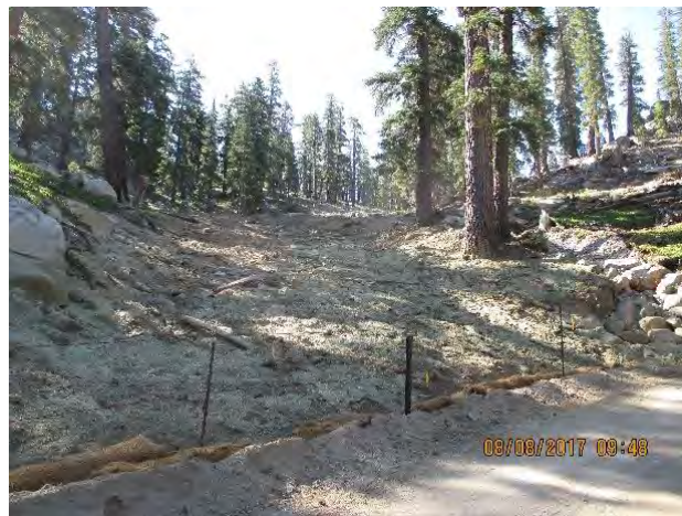
Hand Grenade Chute After: erosion resistance significantly improved on steep slope and toe of slope protection provided by cutoff ditch and pine needle wattle
