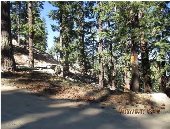
Hand Grenade Chute After: erosion resistance significantly improved on lower road shoulder with pine needle mulch and seed
