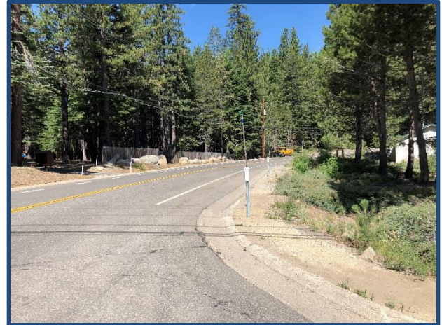
Three-leg stop-control intersection, undivided highway and minor street, no turn storage; North Upper Truckee & San Bernardino Photo: Kittelson
