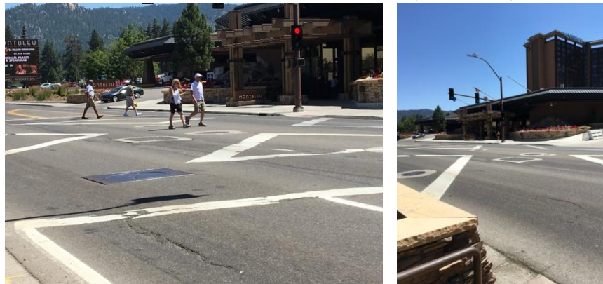
Photo 12- Pedestrian signal head not facing diagonally.
