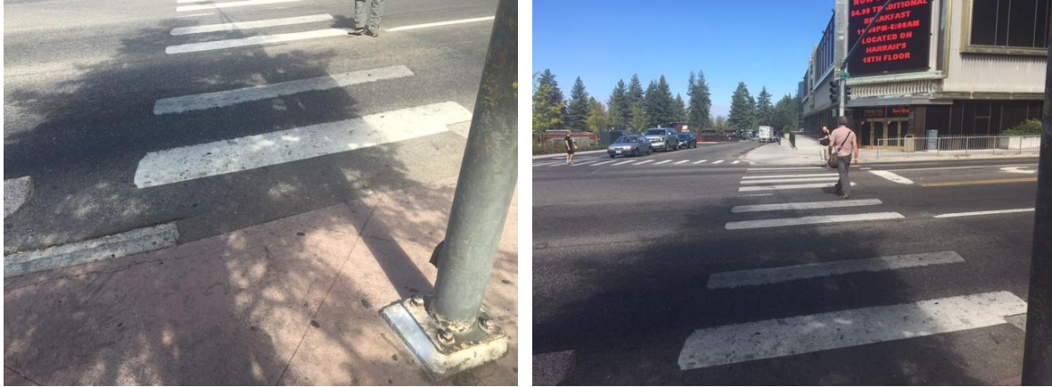
Photo 3- Non-ADA compliant ramps at Stateline.
