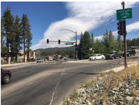
Photo 21- The crosswalk on the intersection of SR 207 (also known as Kingsbury Grade) and US 50 is not in the same line of sight as the driver.
