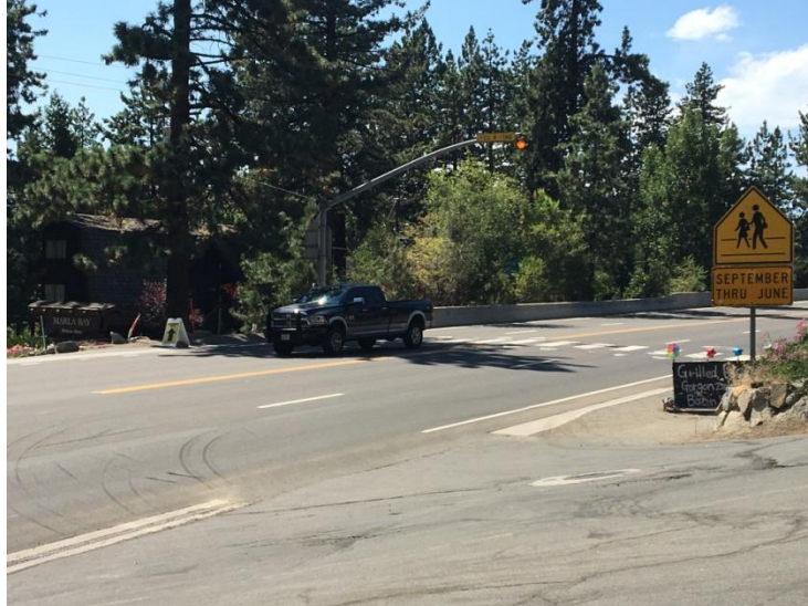
Photo 32- Overhead continuously flashing light.
