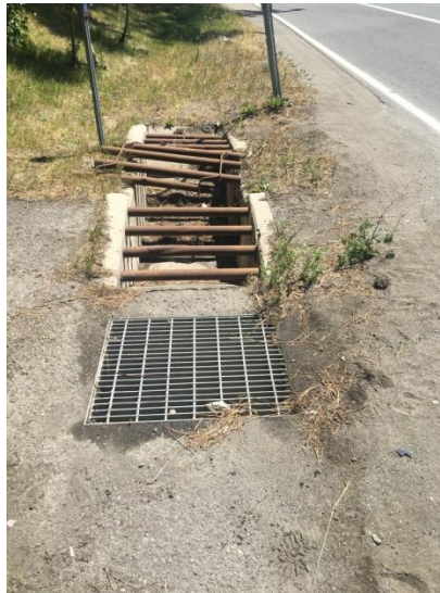
Photo 27- Broken drop inlet.
