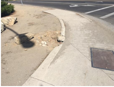
Photo 18-Broken concrete sidewalk.
