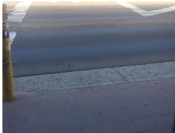
Photo 14- Non-ADA compliant ramp outside CVS lacking detectable warnings.
