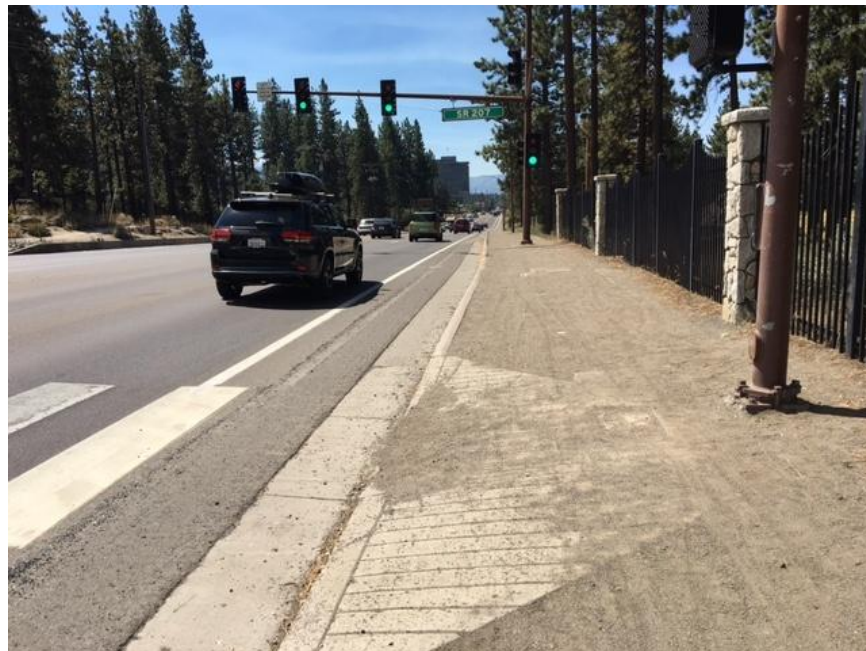
Photo 23- Pedestrian ramp lacking detectable warning.
