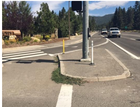
Photo 17-Pedestrian push button at Lake Parkway facing wrong direction and no pedestrian ramp.
