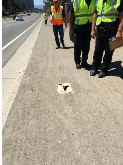
Photo 20- Broken lighting utility box cover.
