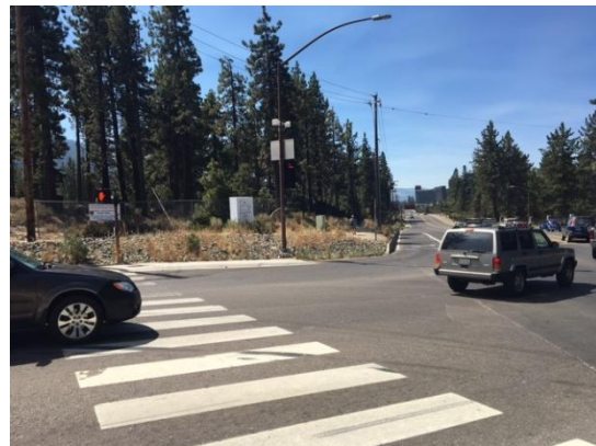
Photo 21- The crosswalk on the intersection of SR 207 (also known as Kingsbury Grade) and US 50 is not in the same line of sight as the driver.
