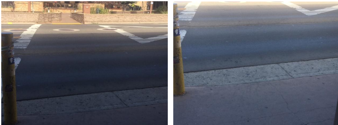
Photo 10- Sidewalks without detectable warning signs
