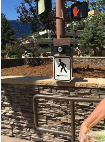
Photo 15-The height of this pedestrian push button outside of Hard Rock Hotel and Casino is non-ADA compliant.
