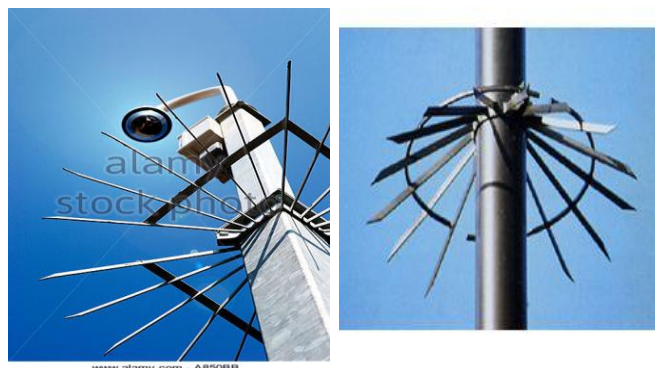
Photo 4- Example of light fixtures used in Las Vegas to discourage pedestrians from climbing.
