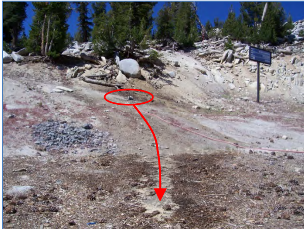
Figure 59. Olympic lift top terminal. Erosion and sedimentation from irrigation. The sprinkler head is circled and the red arrow shows the water flow path.
