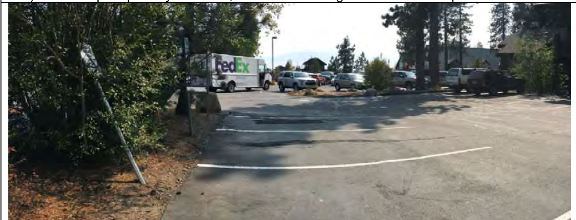
Photo 7 – View south to southwest from northeast corner of APN 094-090-042 (740 N. Lake Blvd.). The north edge of this parcel has a 10-foot high retain wall; parking lot excavated.
