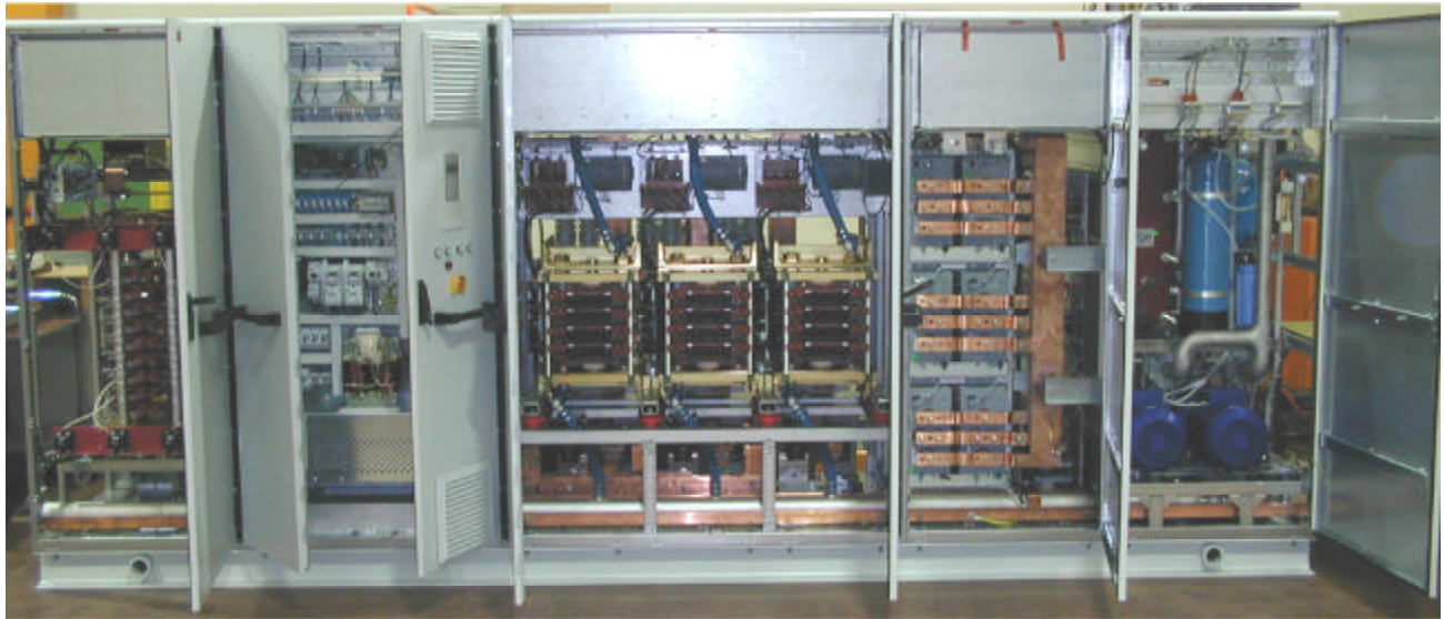
Fig. 5.14: A medium voltage, 3300V IGCT VSI drive for induction motor drives (ABB ACS 6000).
