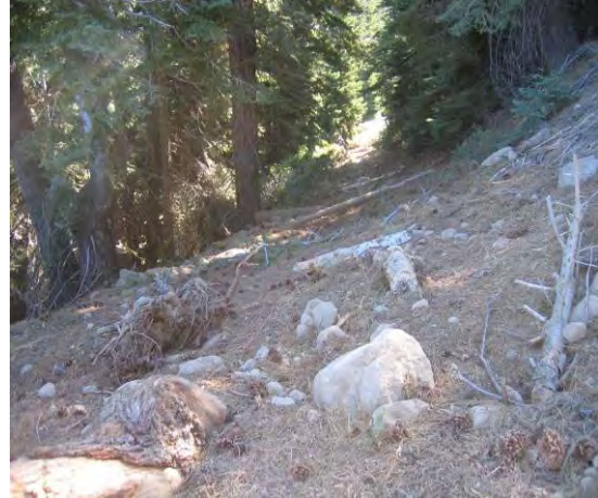
Figure 6. Lower Lombard post-treatment. Slope was re-contoured to match natural slope angle and woody debris and large rocks were added.
