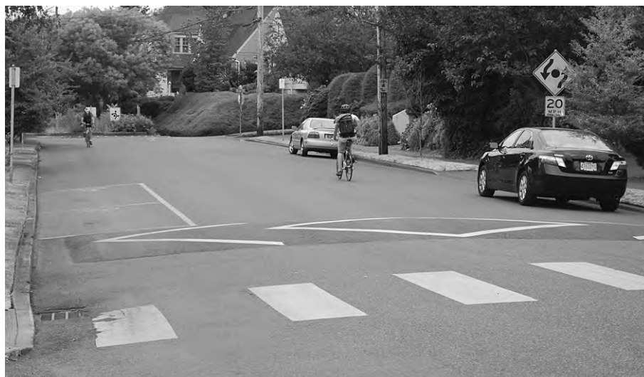
Fig. 3. Bicycle boulevard in Portland, OR with speed hump and traffic circle to slow and divert motor vehicles (photo by J. Dill).
