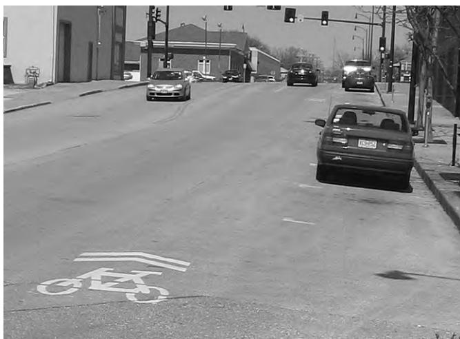
Fig. 4. Shared lane marking in Columbia, MO (photo by J. Dill).
