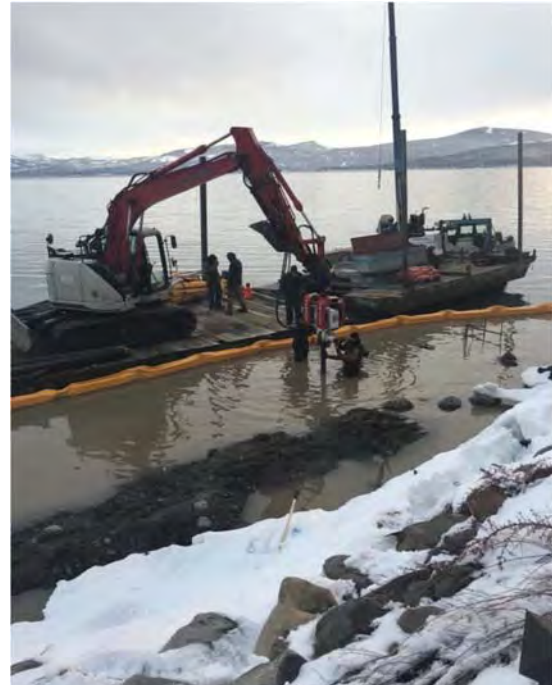
Initial pile driving for pipe anchor supports.
