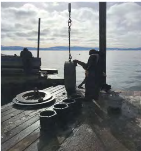
Placing and adjusting temporary manhole risers.
