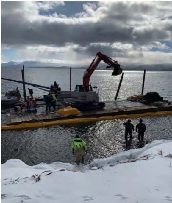
Initial mobilization and installation of turbidity curtain.
