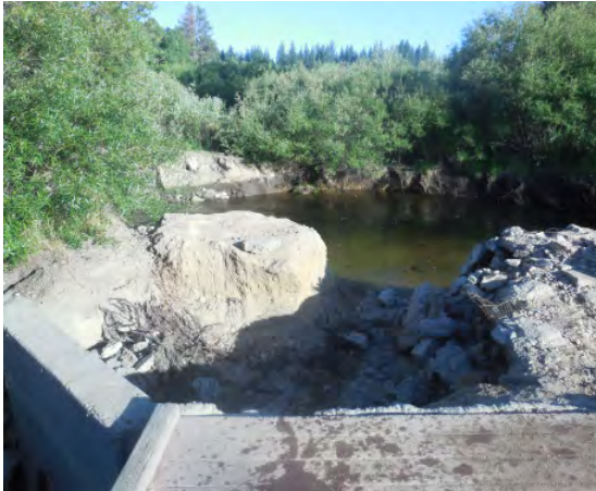
Summer 2017, bridge not connected to West side
