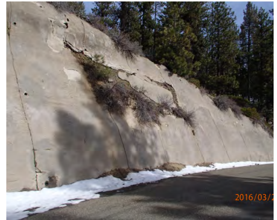
Oflyng - Failing Slope
