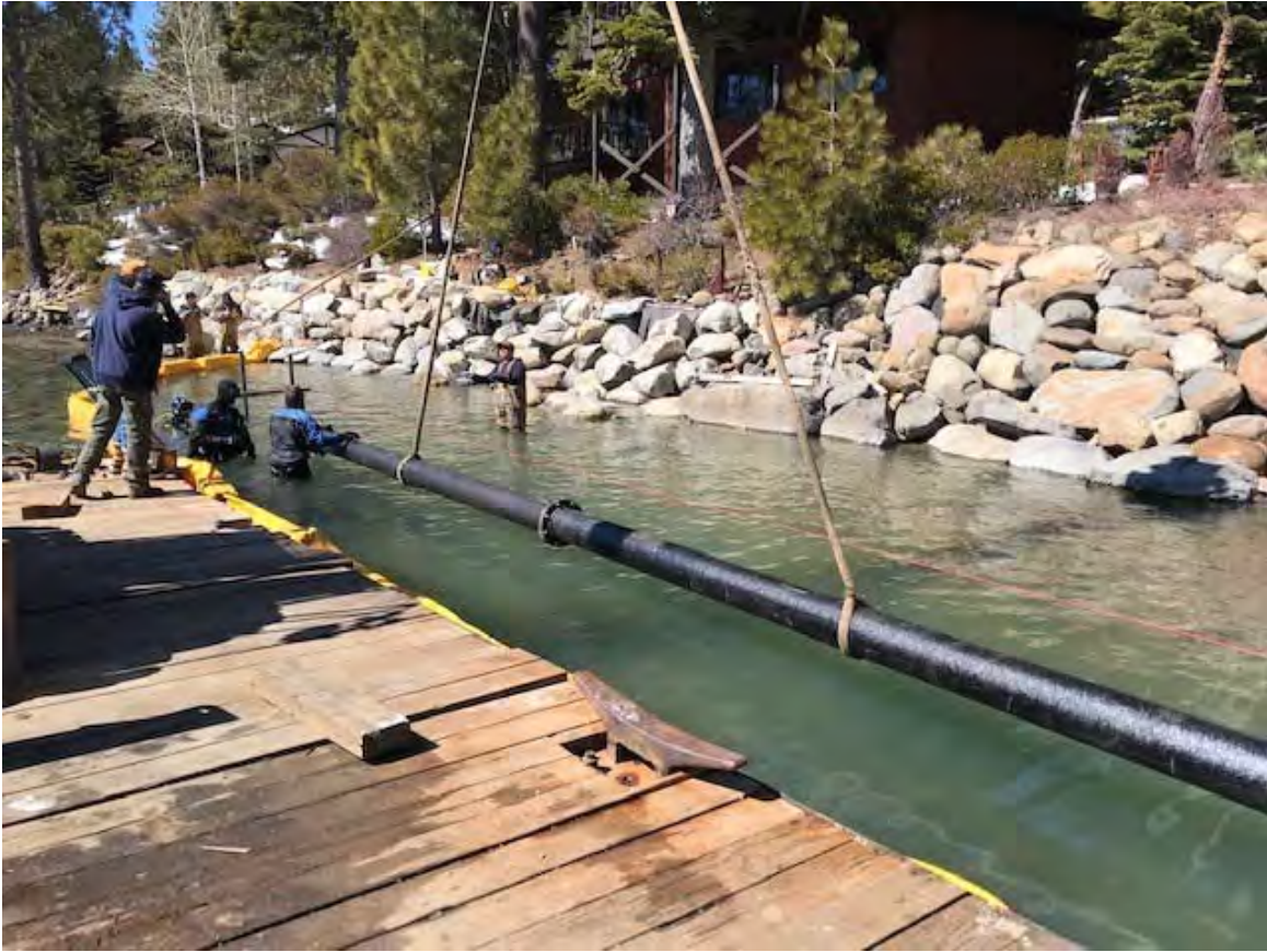
Fig. 12 – D.I.P. installation.
