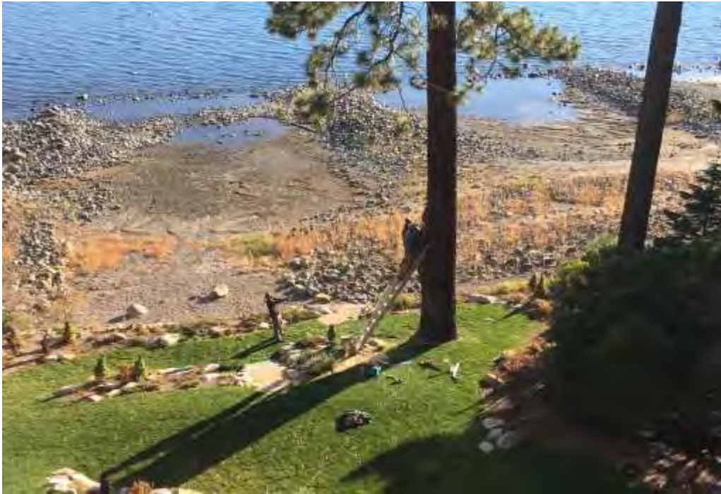
Appellants' Beach on 11/5/2015 Showing Sewer Pipe Completely Buried
