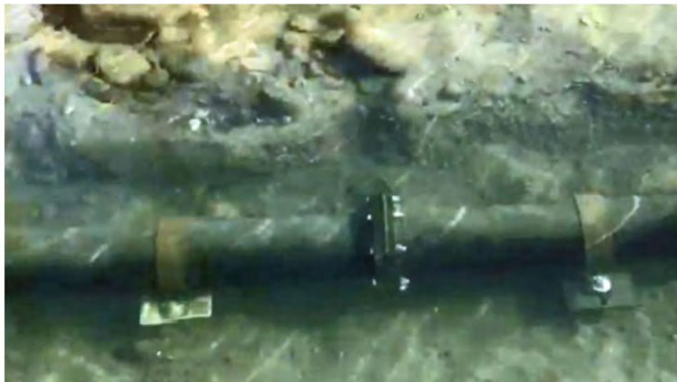
Pipe in place.
