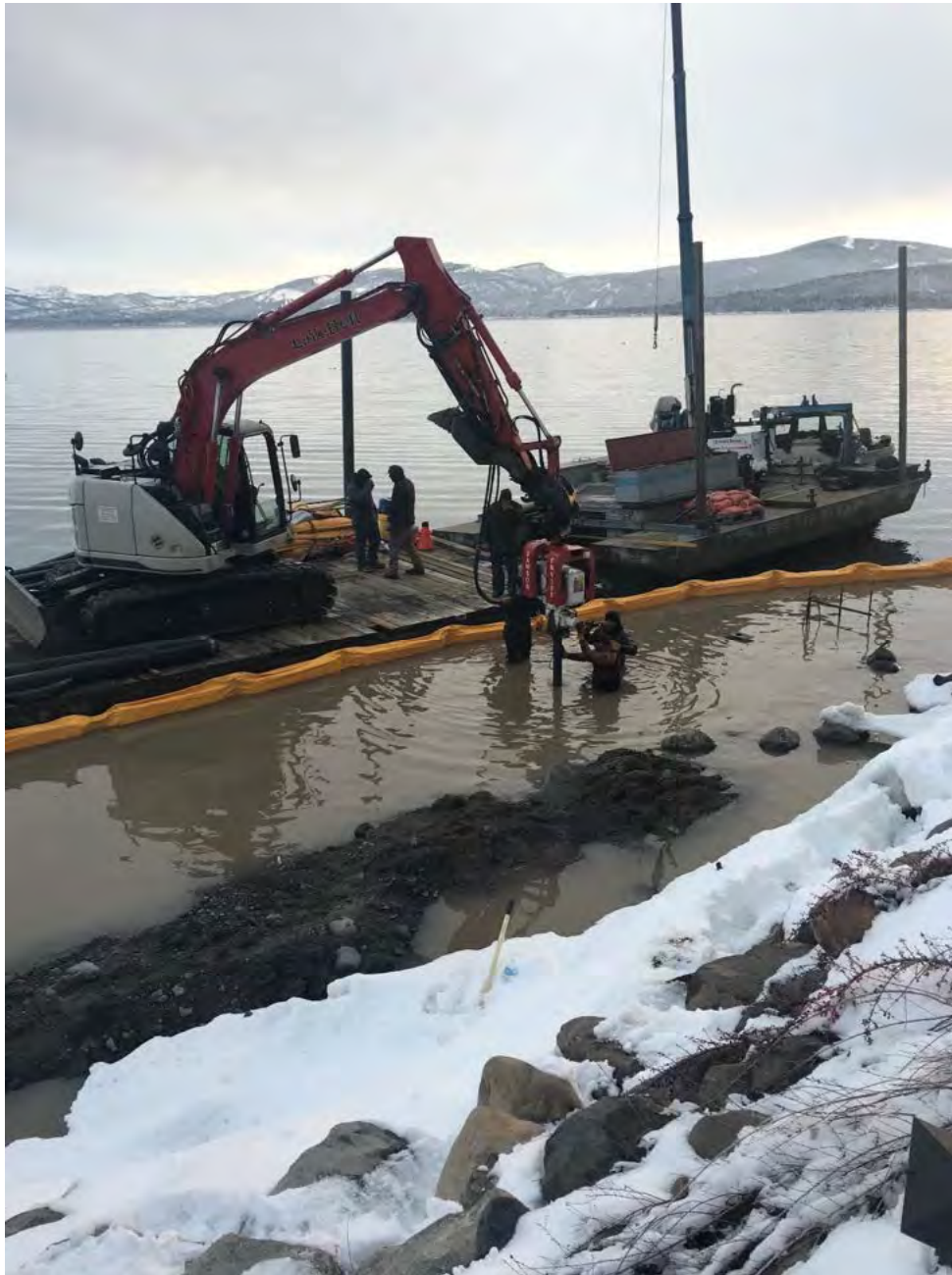
Fig. 6 – Initial pile driving for pipe anchor/supports.
