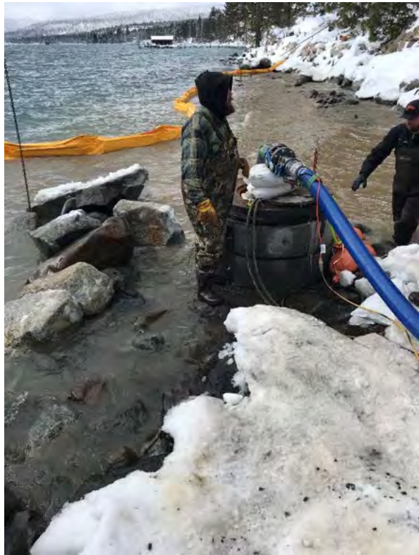
Fig. 3 – Adjusting manhole risers (Feb. 8 th ).
