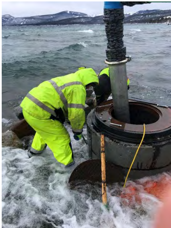
Fig. 4 – Fastening risers in place (Feb. 12 th ).
