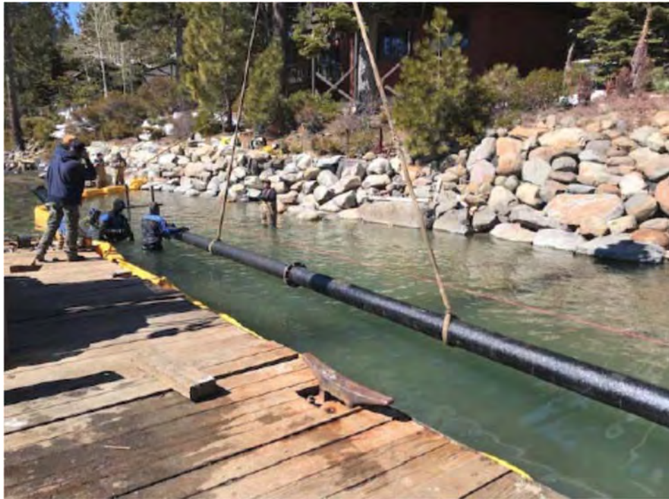
Maneuvering pipe into position.
