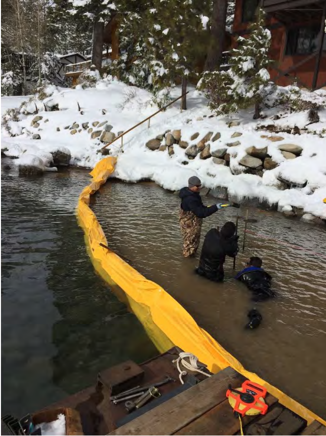
Photo 4 – Turbidity curtain around downstream end of pipe repair. .
