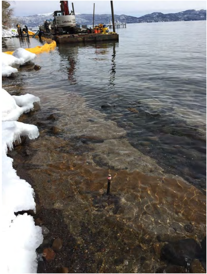
Photo 5 – Trench excavation through volcanic ash.
