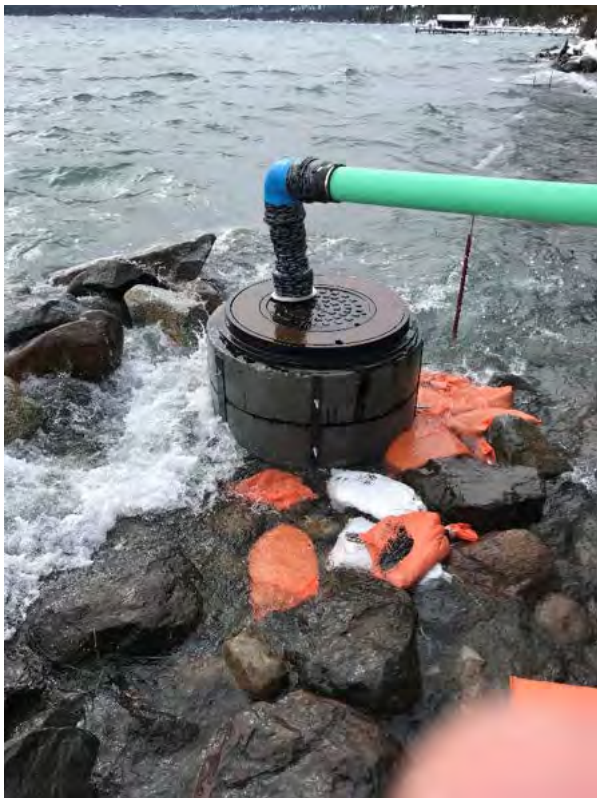
Fig. 5 – Complete temp. riser installation (Feb. 12 th ).
