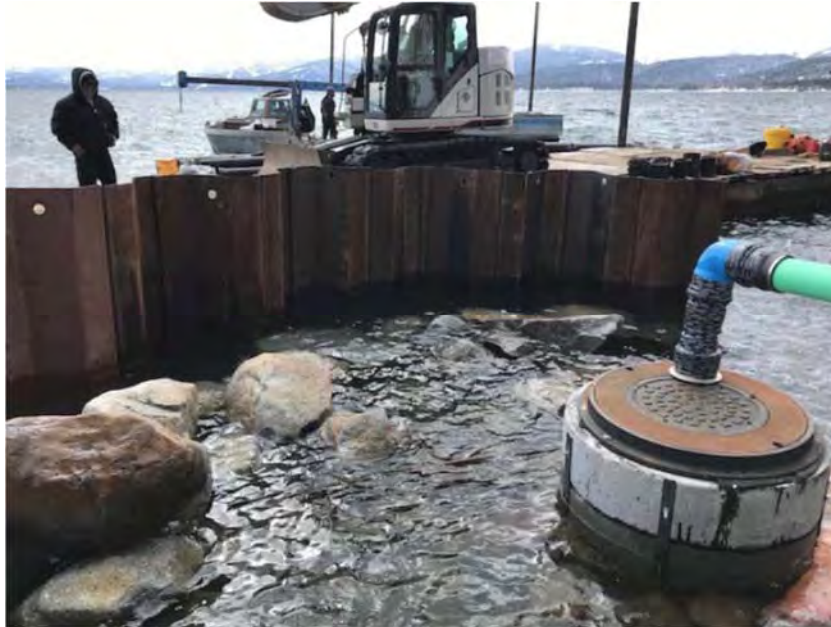
Sheet piling installed near sewer manhole.
