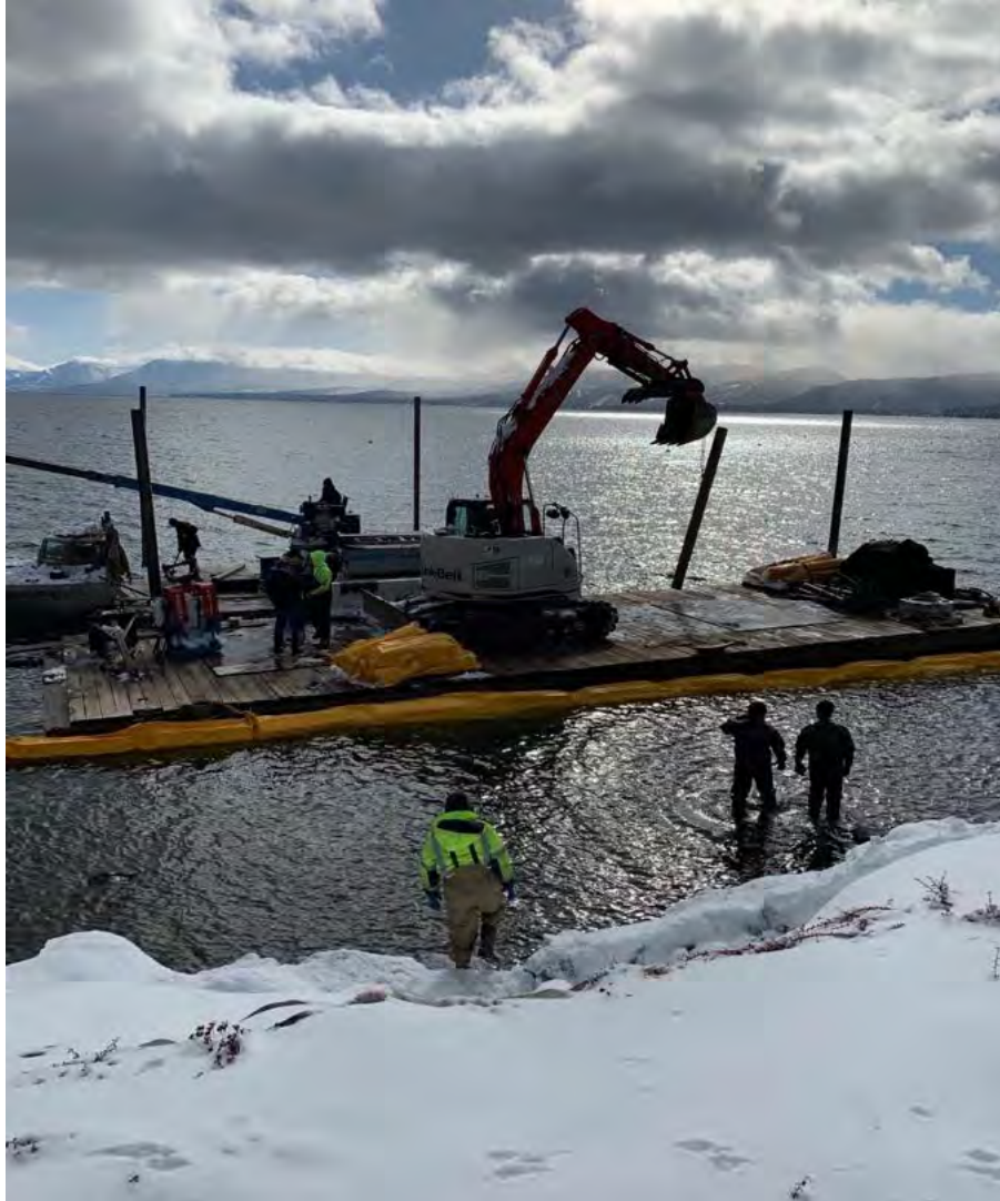
Fig. 1 - Initial mobilization and installation of turbidity curtain.
