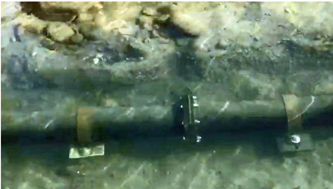
Fig. 13 – Completed pipe installation.
