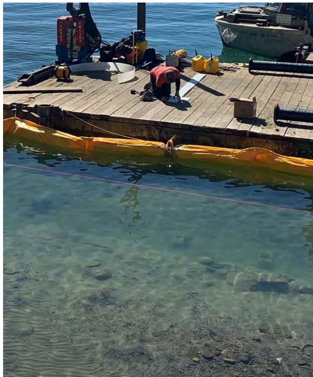
Fig. 10 (above) verifying anchor/support grades & Fig. 11 (below) pile driving completed.
