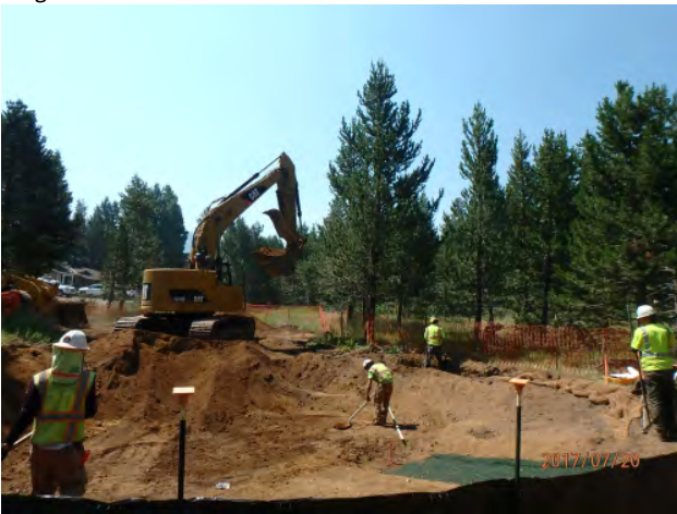
Construction of infiltrating sediment basin.
