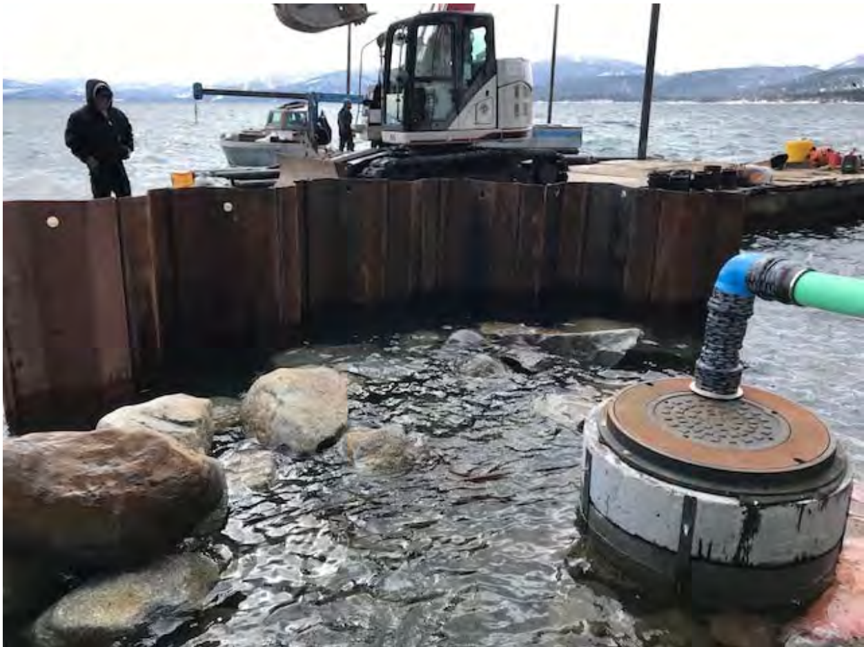
Fig. 7 – Sheet piling installed near sewer manhole Sta: 17+65.
