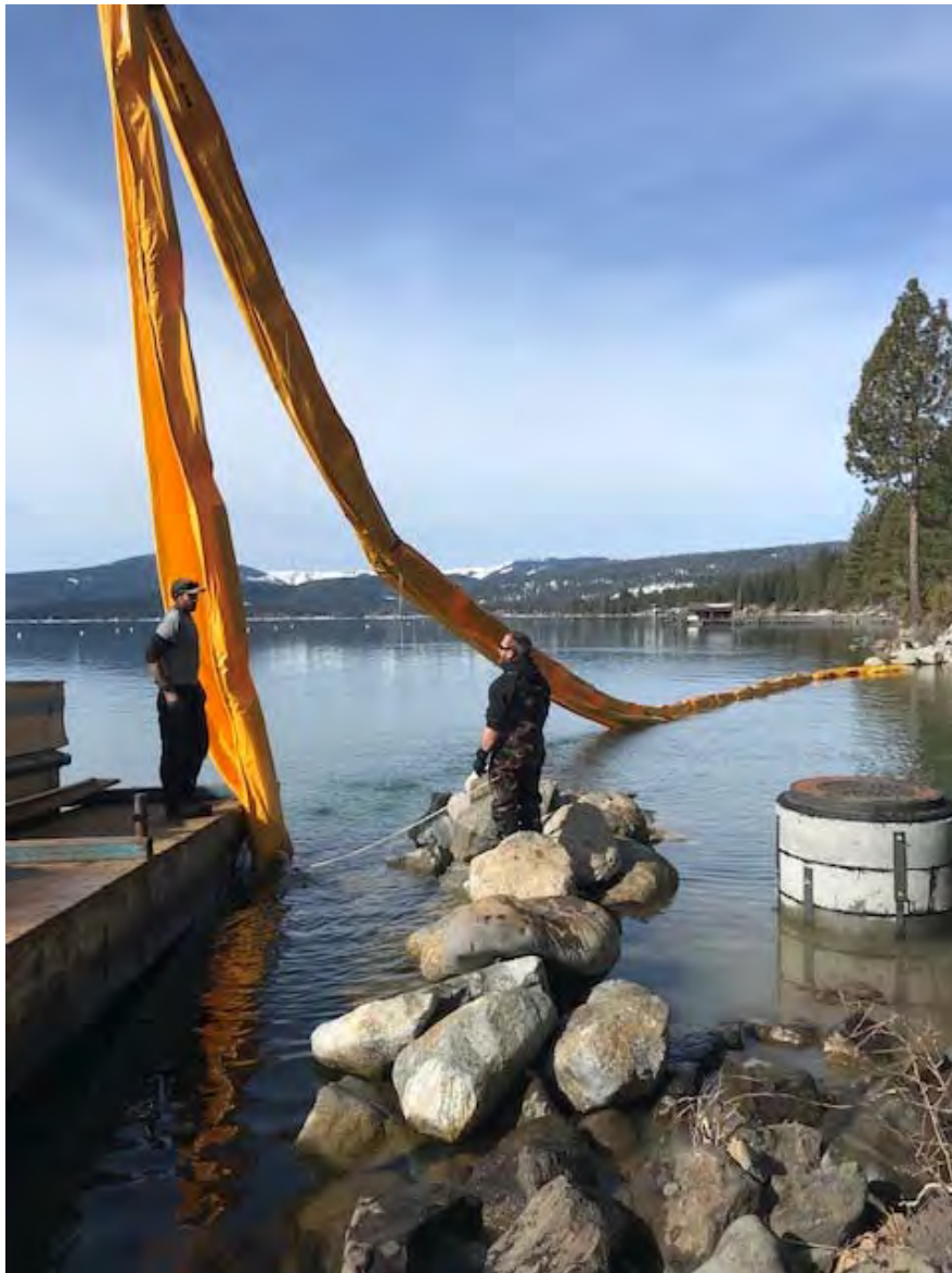
Fig. 14 – Removal of turbidity curtain. (March 19 th , 10:30 am)
