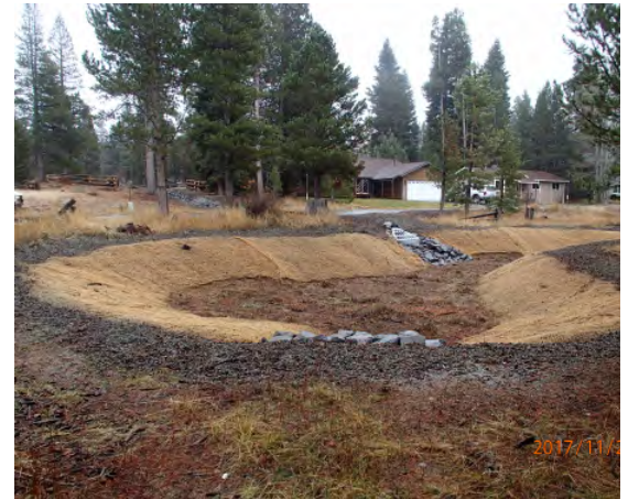
Completed infiltrating sediment basin.
