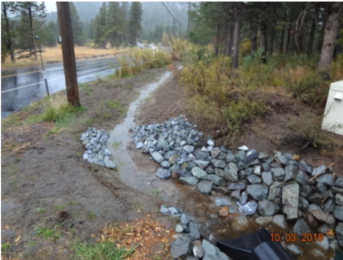
New channel on east side of lower Elks Club Drive
