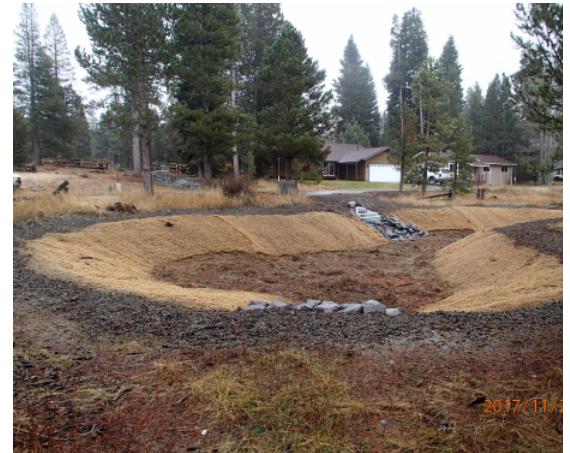
Completed infiltrating sediment basin.
