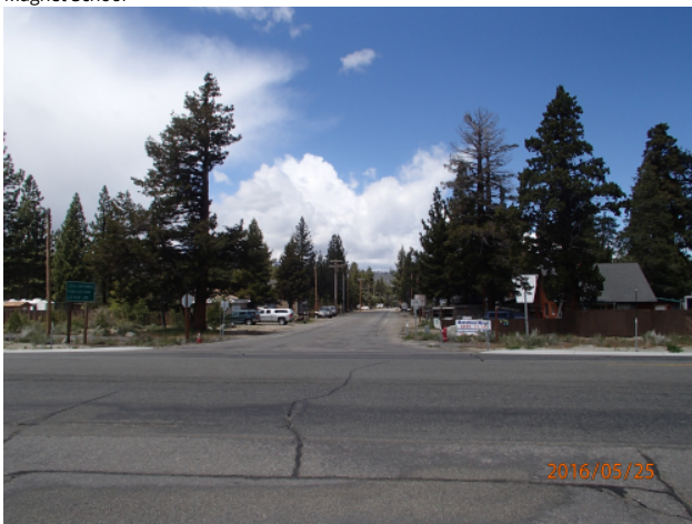
view to the north at the Apache Ave intersection, from US 50/SR 89
