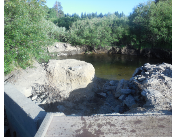
Summer 2017, bridge not connected to West side
