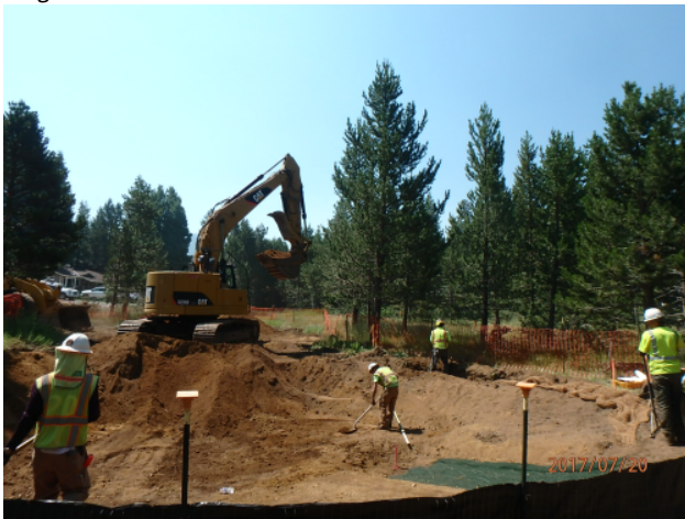
Construction of infiltrating sediment basin.
