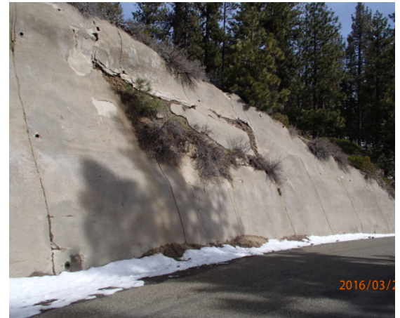
Oflyng - Failing Slope
