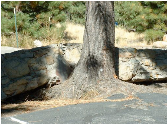
Pine abutting stone wall, lifting asphalt.
