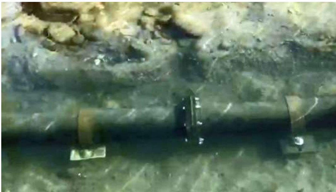
Figure 13, TCPUD NOC to Army Corps of Engineers – Replacement Pipe in Trench
