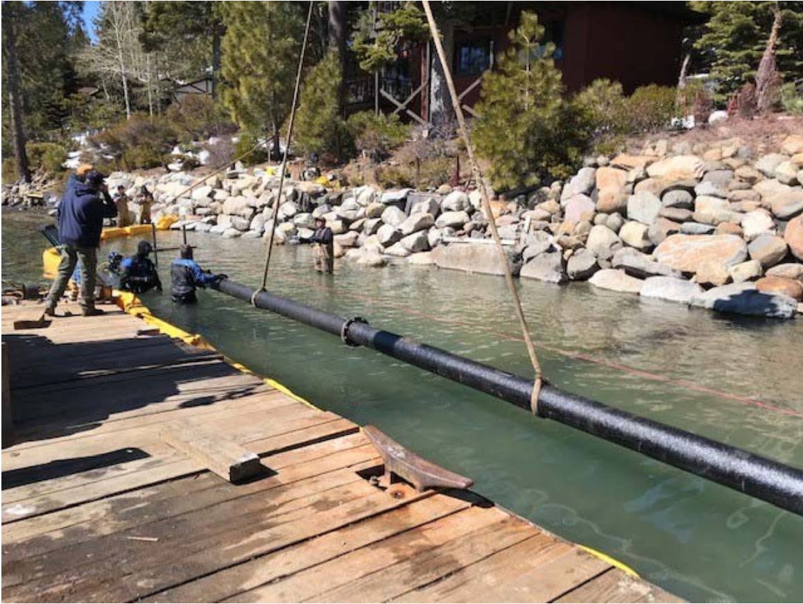
Fig. 12 – D.I.P. installation.
