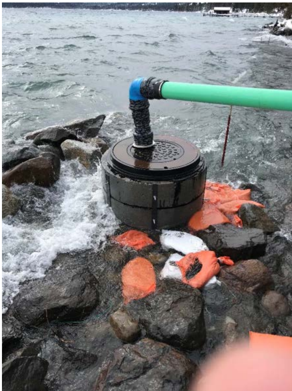
Fig. 5 – Complete temp. riser installation (Feb. 12 th ).
