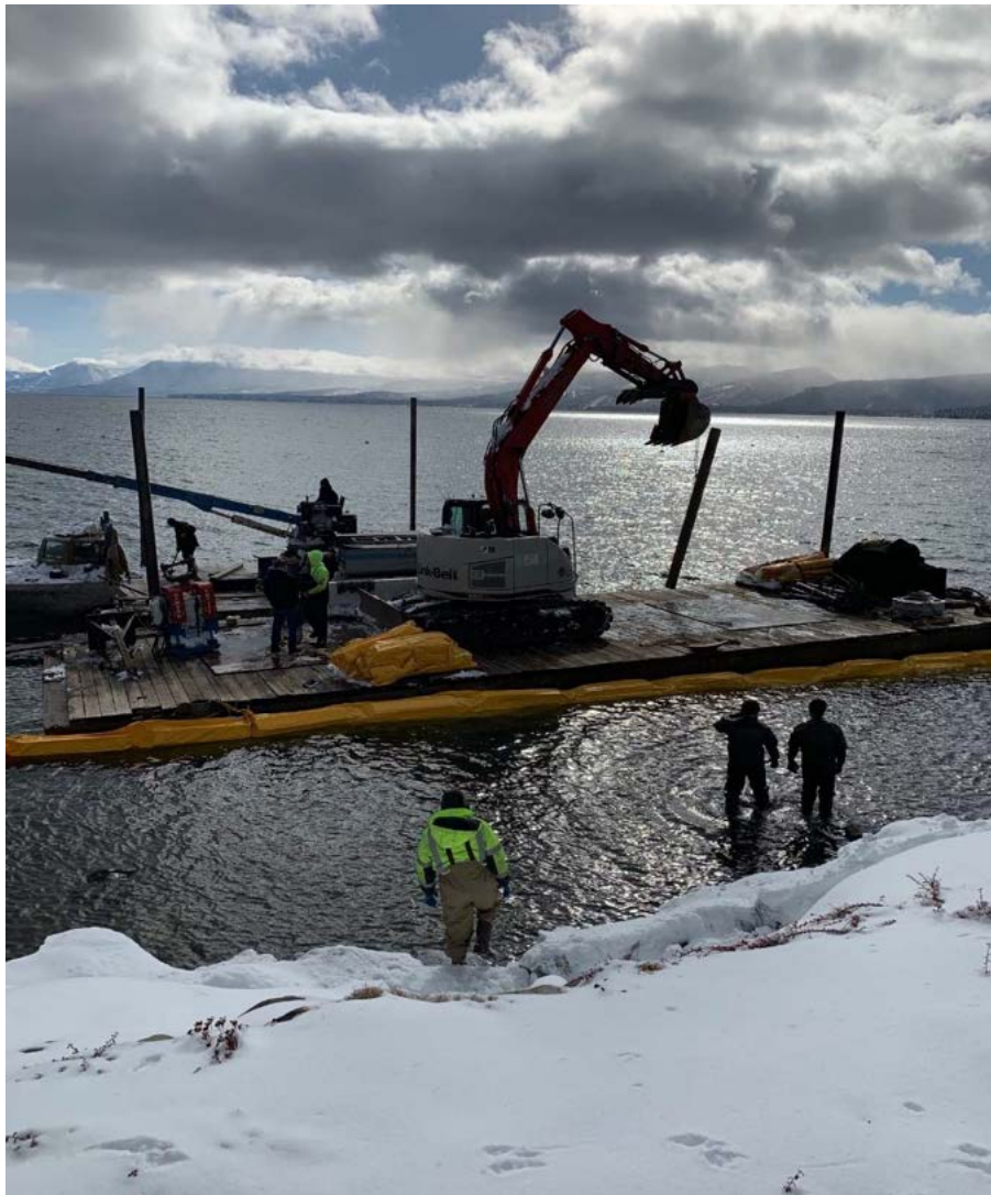
Fig. 1 - Initial mobilization and installation of turbidity curtain.
