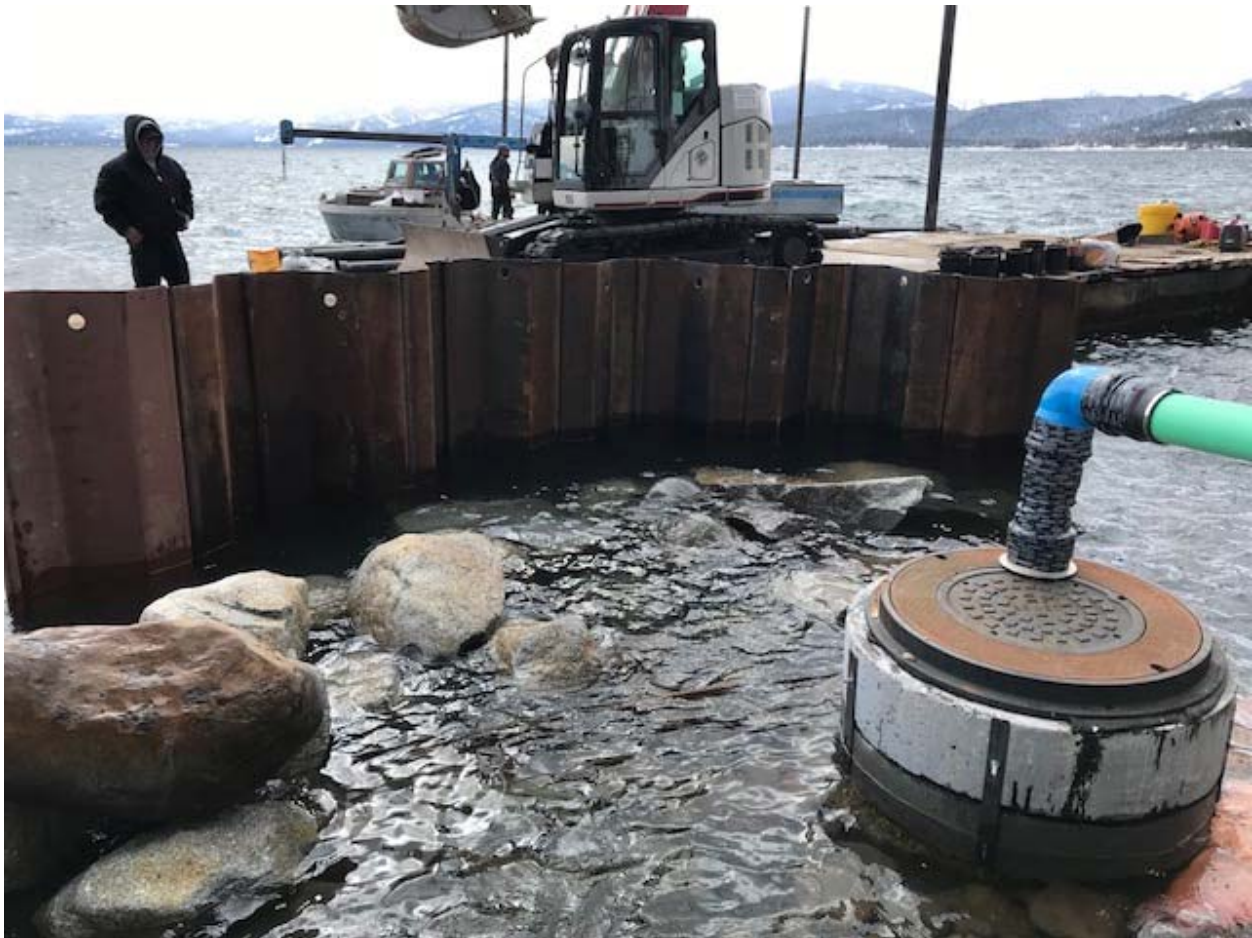
Fig. 7 – Sheet piling installed near sewer manhole Sta: 17+65.
