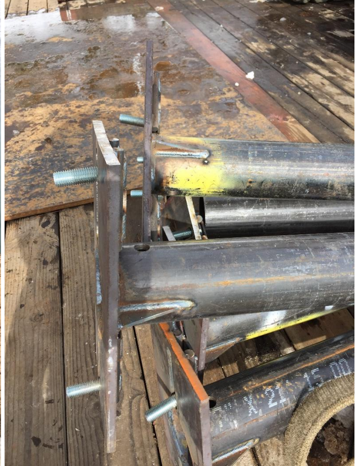
Photos 2 and 3 - Pipe Piles with ½-inch plate welded to top where hold-down strap will be bolted to hold pipe.
