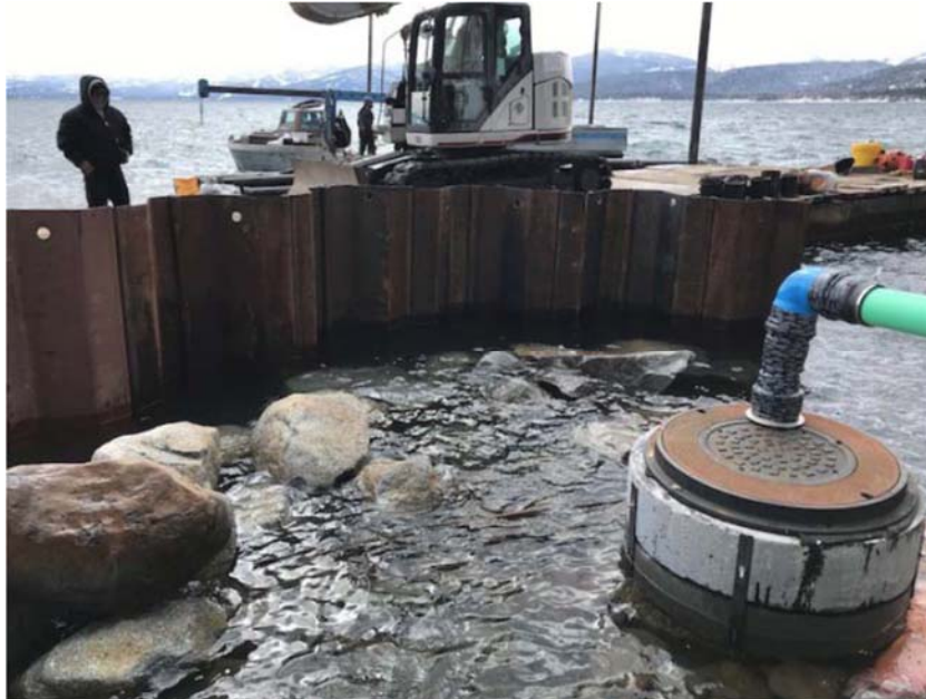
Sheet piling installed near sewer manhole.
