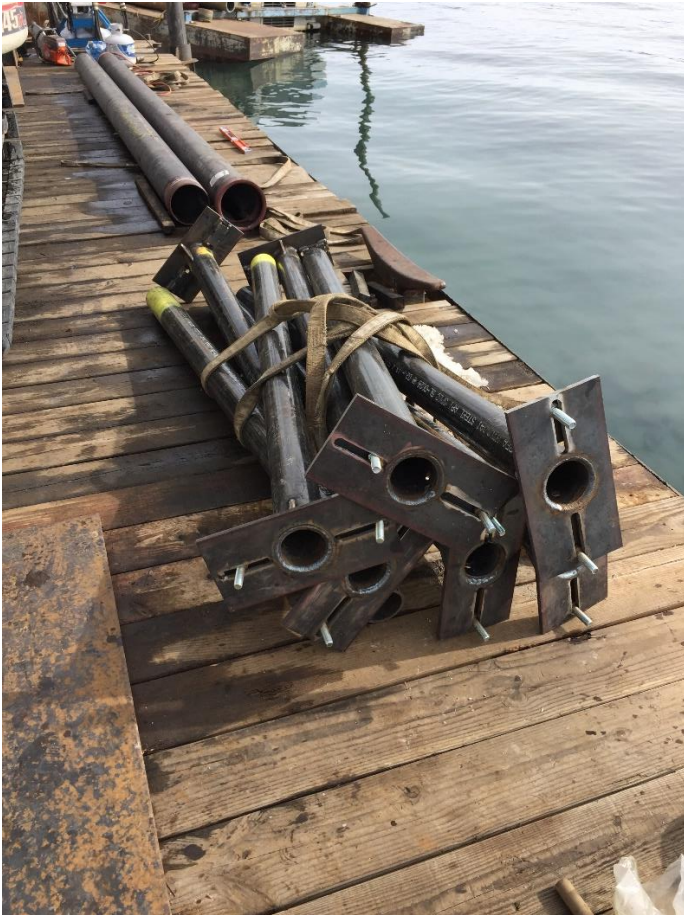
Photos 2 and 3 - Pipe Piles with ½-inch plate welded to top where hold-down strap will be bolted to hold pipe.
