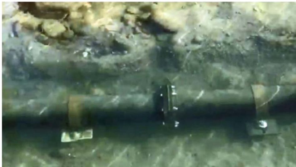
Pipe in place.
