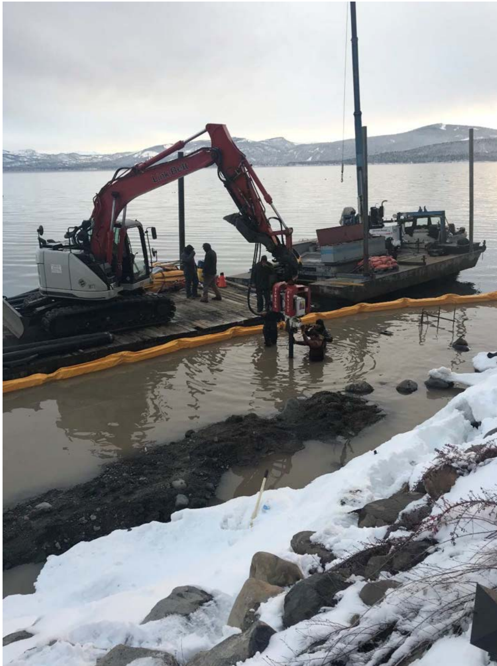
Fig. 6 – Initial pile driving for pipe anchor/supports.
