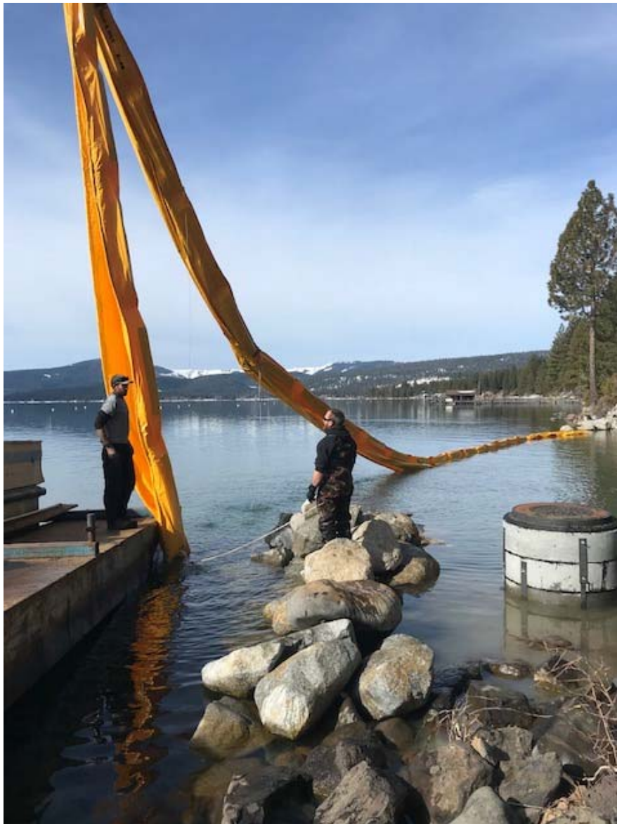
Fig. 14 – Removal of turbidity curtain. (March 19 th , 10:30 am)
