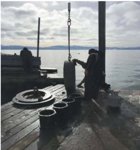
Placing and adjusting temporary manhole risers.
