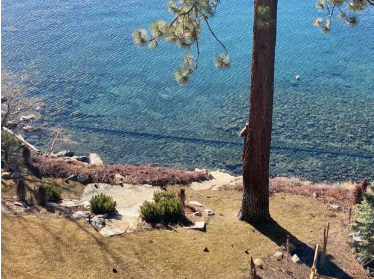
Exposed Sewer Pipe 1/20/2020
