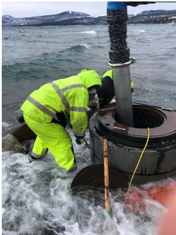
Fig. 4 – Fastening risers in place (Feb. 12 th ).
