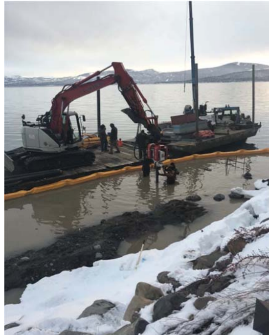
Initial pile driving for pipe anchor supports.
