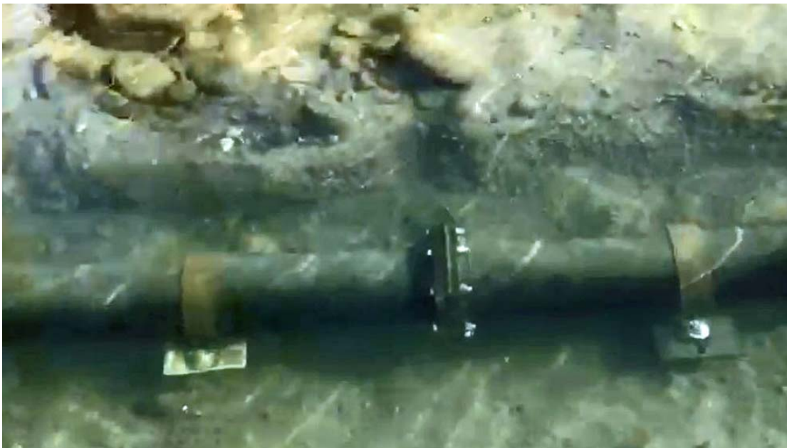
Fig. 13 – Completed pipe installation.
