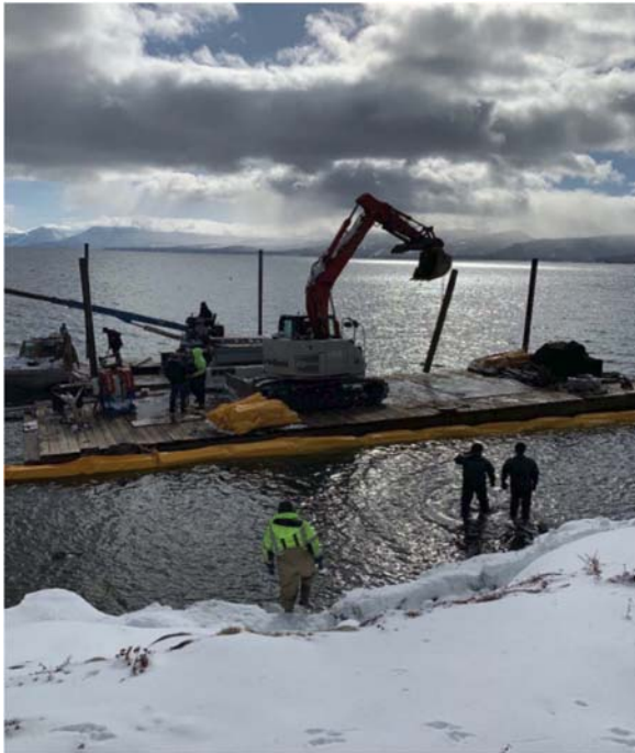
Initial mobilization and installation of turbidity curtain.
