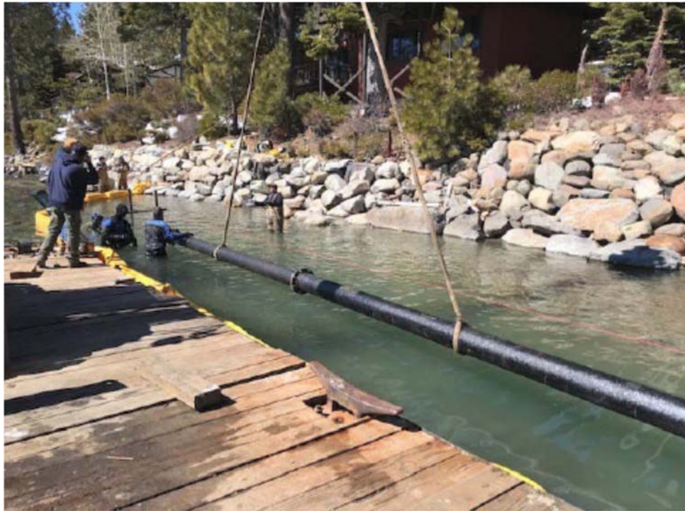
Maneuvering pipe into position.
