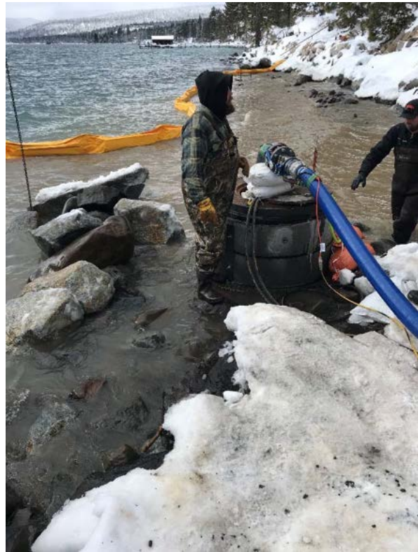
Fig. 3 – Adjusting manhole risers (Feb. 8 th ).
