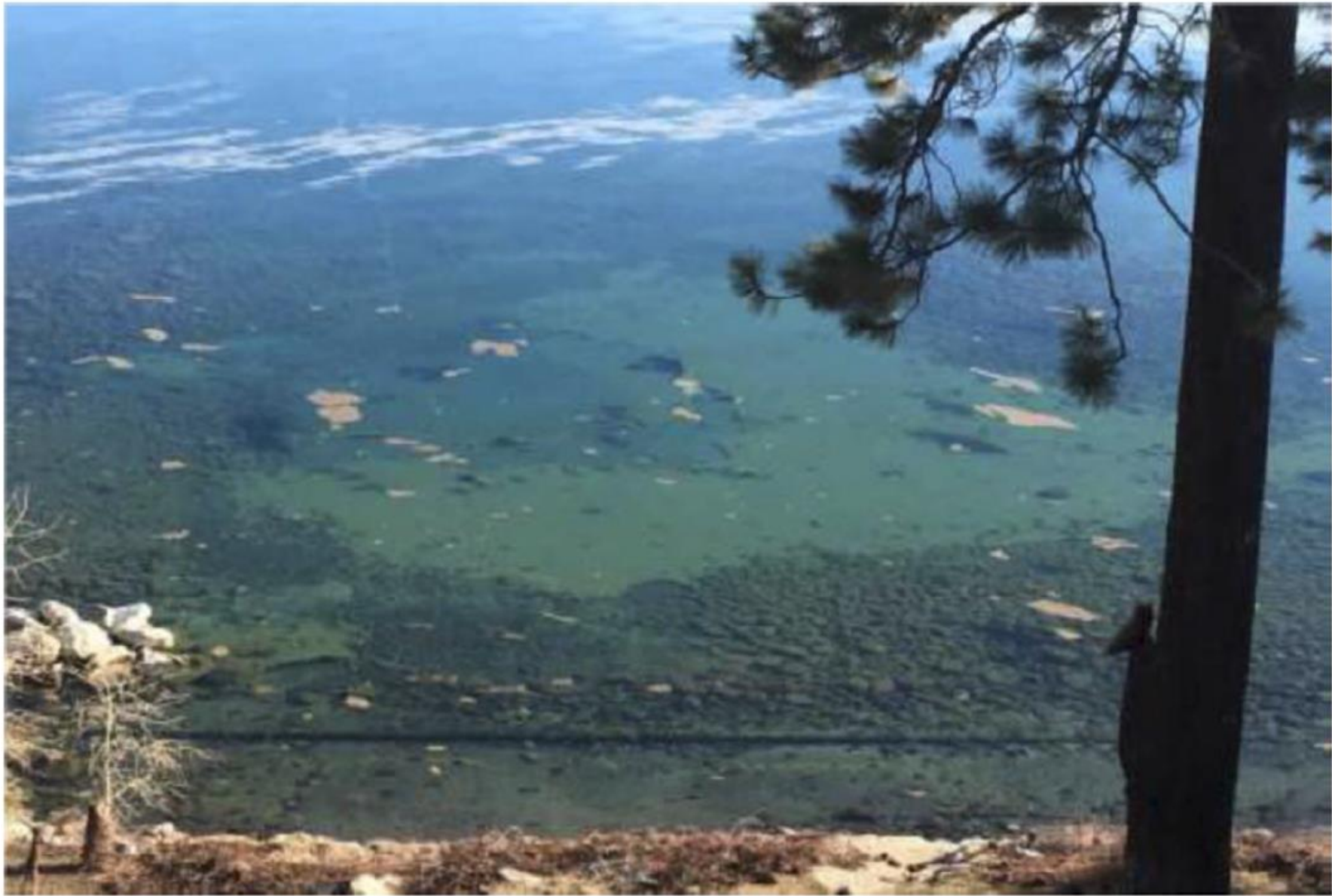
Exposed Replacement Pipe Photographed on 3/31/2019 – Twelve Days After Completion
