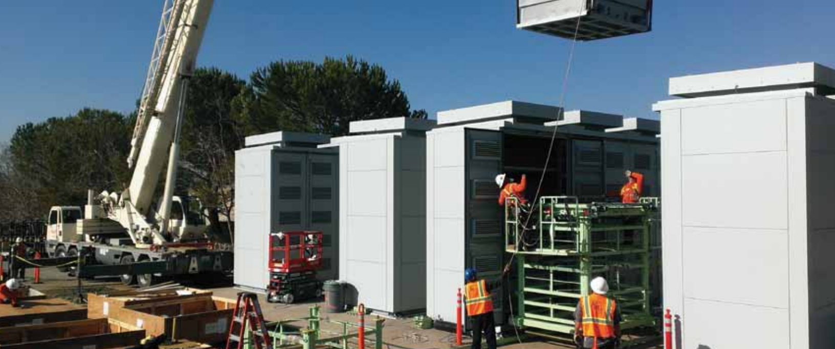
Battery modules being loaded into cabinets at PG&E's NaS battery system installation underway in San Jose
