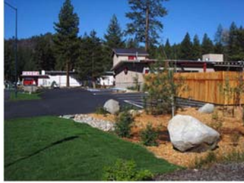
Ensure that loading areas do not interfere with other site circulation, and permit free use of aisles, driveways, and sidewalks during freight operations.
